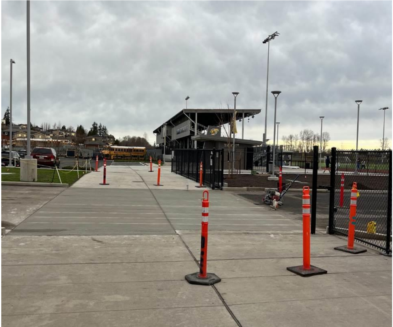
The completed new sidewalk crossing
