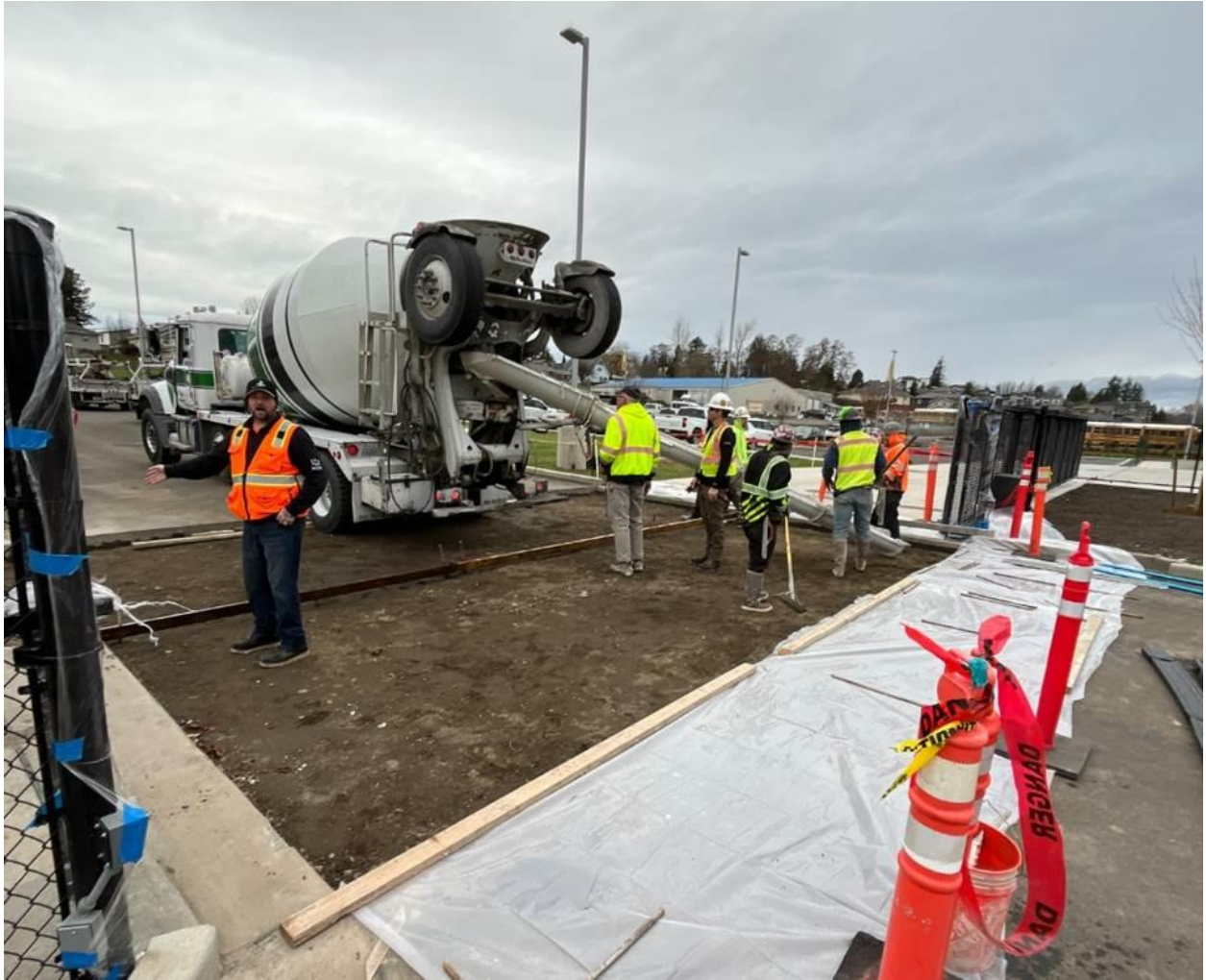
Crews pouring the final sidewalk crossing near Golden Eagle Stadium
