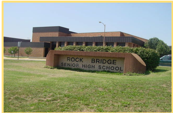
Rock Bridge High
