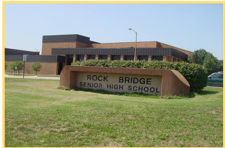
Rock Bridge High
