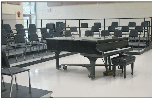
The music rooms at Brentwood High School were cleaned and renovated with new flooring.
