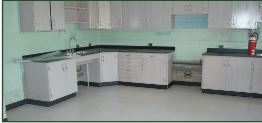
New cabinetry and asbestos abatement were both part of the undertaking at North Middle School.
