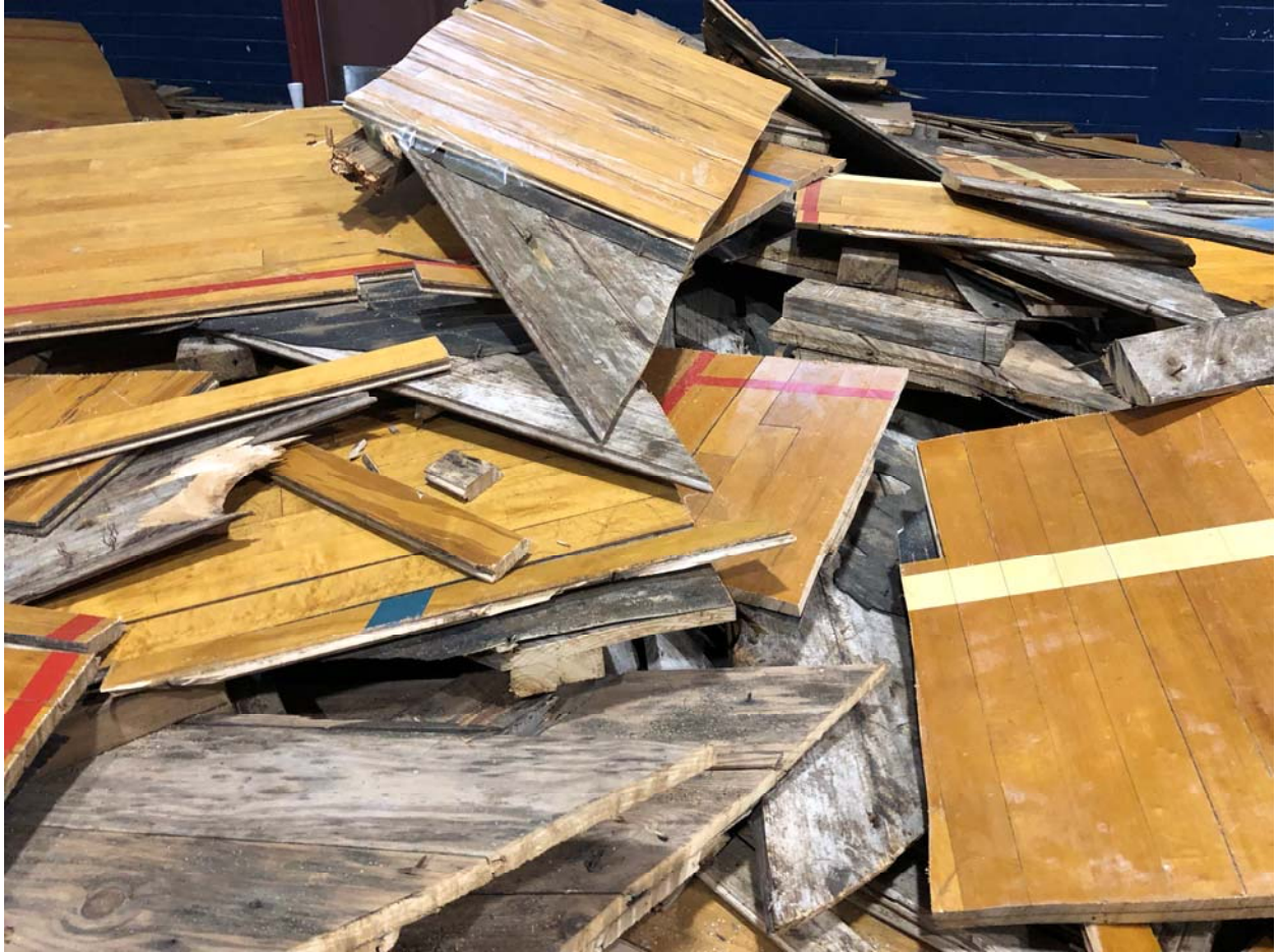
Gym Floor Demolition Debris
