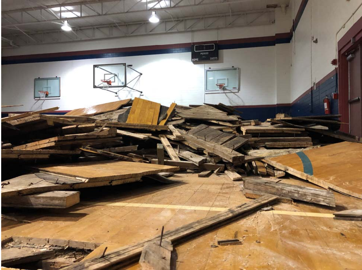
Gym Floor Demolition Debris
