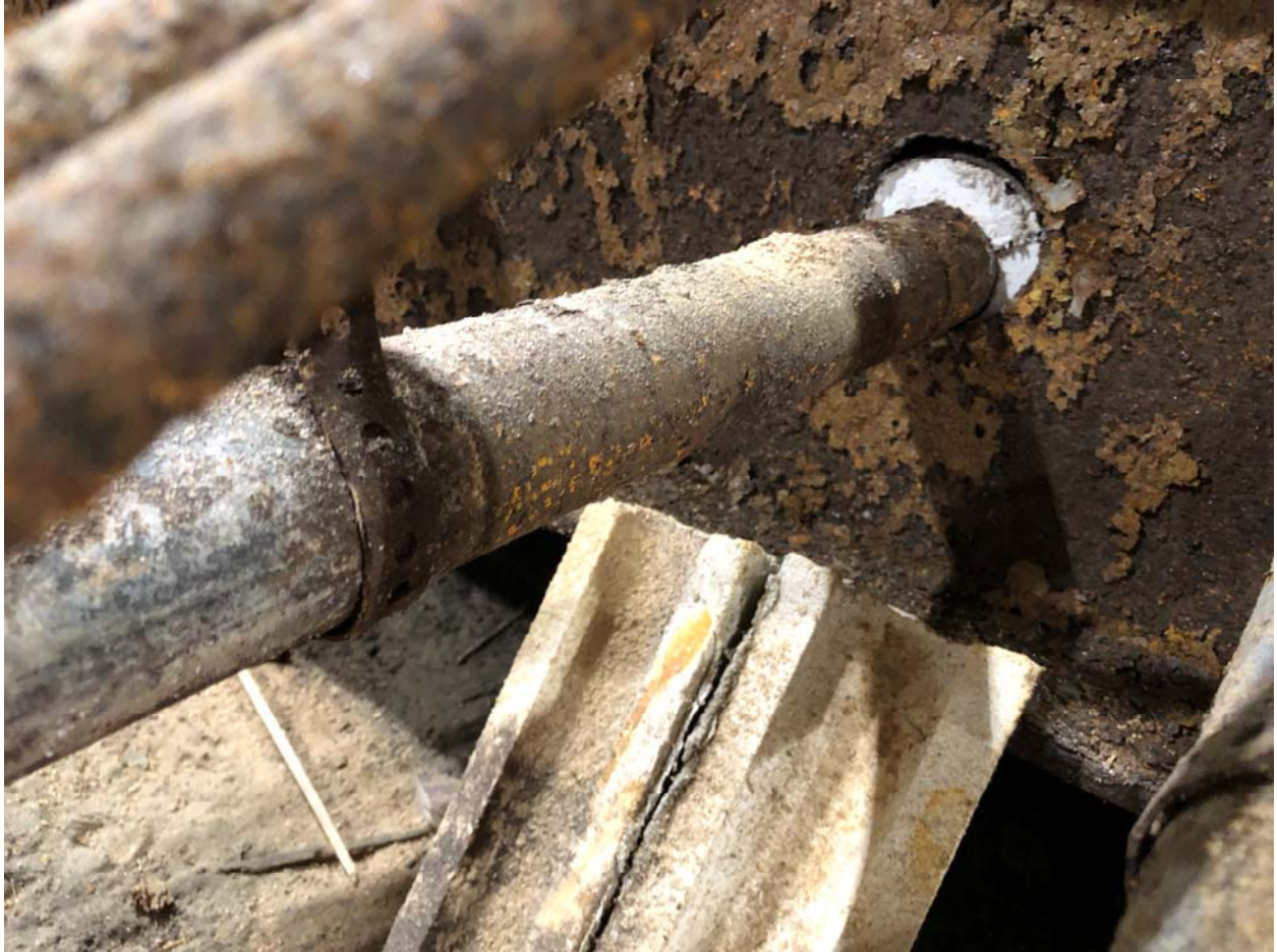
Crawlspace Pipes Penetrating Beam
