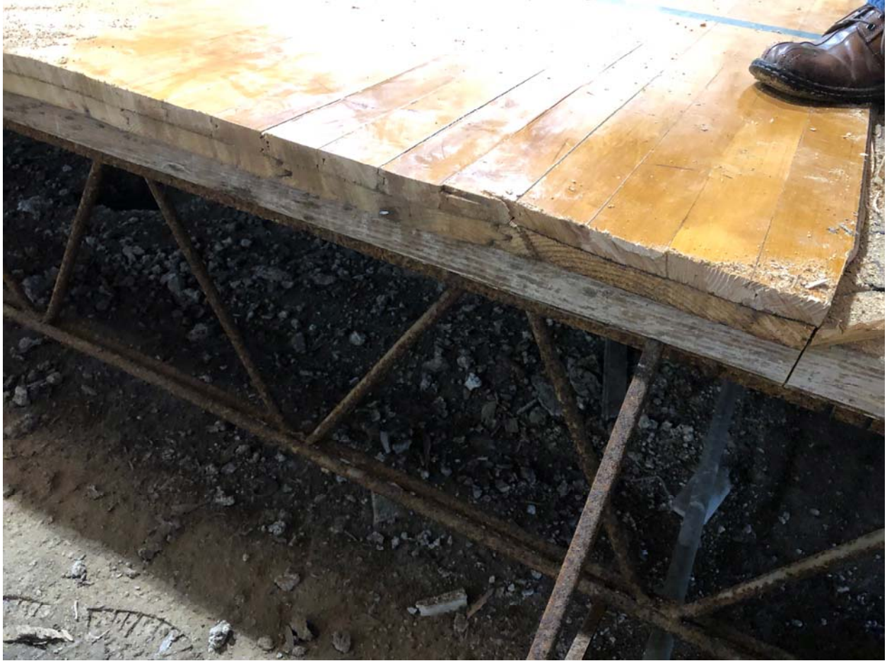
Gym Floor and Crawlspace
