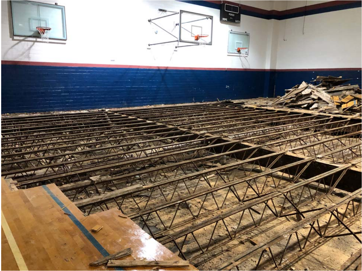
Partially Demolished Gym Floor and Crawlspace
