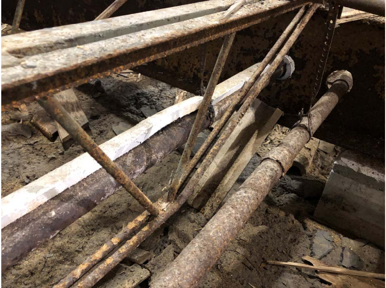
Crawlspace Pipes Penetrating Beam
