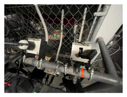
Various boxes for rehearsal lights, DMX, and dimmer power are located throughout the catwalk area, but they disorganized and do not provide a coherent circuiting layout for lighting fixtures.
