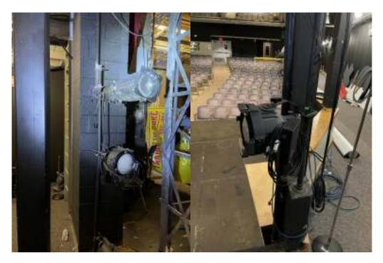
**Recommendation:** These positions should be replaced with properly fabricated single units with welded components and mounted to the floor.
