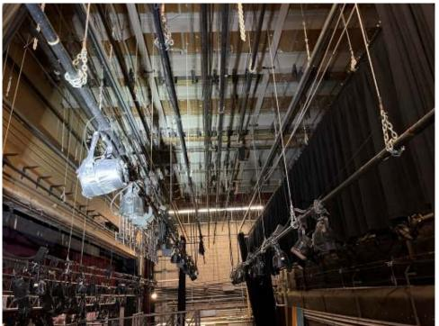
**Recommendation:** Replace the distribution, cable management and multicable with new full length connector strips, providing additional circuits and DMX control across the length of the pipe. If the intent is to motorize these electrics, provide hoist systems with integrated cable management.
