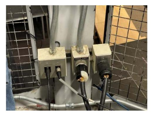
Many areas have dimmer bars that are not mounted. Many of the dimmer bars are located in areas that could be considered unsafe, either in terms of access to those areas or in terms of positioning to maintain safe operation and space for heat dissipation.
