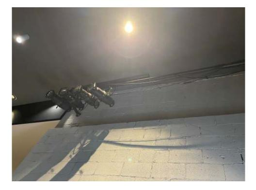
**Recommendation:** The front of house positions could be remounted lower for easier access. Refabricate new torm pipes with welded corners and flanges. Permanent power and control wiring should be installed.
