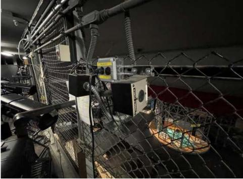
**Recommendation:** The catwalk power and control distribution should be reorganized and replaced. New outlet boxes and DMX outlets should be mounted at locations across the catwalk to minimize extra cabling.
