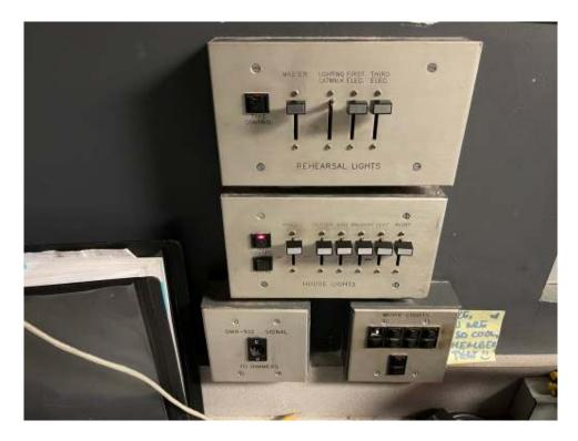
Some house light fixtures are not connected to the lighting system at all, and therefore not controllable for performances. Many of the house light fixtures need new lamps. A pendant fly system is required to reach some of the fixtures for re-lamping.
