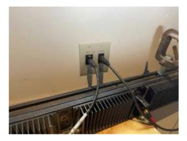
**Recommendation:** Update DMX control distribution system to modern networking equipment and cabling. Provide control locations at all fixture hanging positions. Control locations should be addressable to facilitate system setup.
