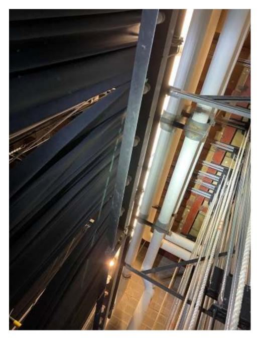
**Recommendation:** Work lights should be provided on the electrics for lighting the stage area to build scenery, etc. Additional high work lights to enable visibility of the rigging would also be an improvement. Replace and /or repair work lights on the catwalk and in the tech galleries. Index lights on fly rail need replacement lamps or should be updated to LED.
