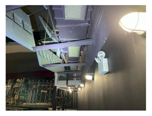
**Recommendation:** The house light system should be replaced in its entirety, with the dimmer units replaced by relay panels. The house lighting fixtures should be replaced with DMX controlled LED fixtures, uniform in type throughout the space to provide adequate levels of light to maintain safe egress. Pendant winches should no longer be needed, as lamp replacement should be minimal.
