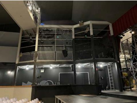
**Recommendation:** Dimmer bars should be replaced with permanent power and control wiring at multiple locations to minimize cabling all over the position.
