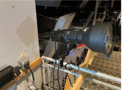
**Recommendation:** Lighting fixtures are clamped to balcony guard railing and should be mounted on follow spot stand pipe. Permanent power and control wiring should be provided. Upgrading fixtures upgraded to LED will no longer require a separate dimmer. City Theatrical offers a follow spot kit for more stable mounting, handling, and balance of the fixture.
