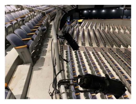
**Recommendation:** A separate hanging position could be created 6 or 8 Inches out from rail so lights could be hung in proper orientation with the yoke mounted vertically, to keep lighting fixtures away from the audience area and out of audience sight lines. Permanent conduit and circuit boxes should be run out to the new hanging positions.
