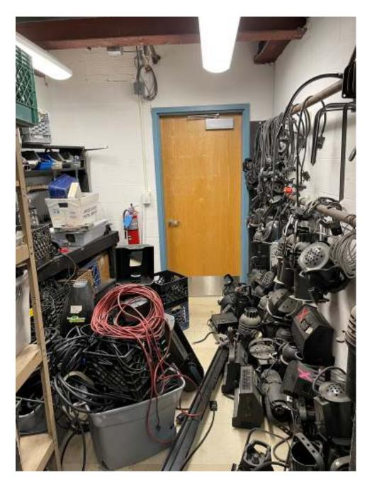
**Recommendation:** Replace all of the non-LED fixtures with new LED fixtures. Add some automated lighting fixtures. Provide new cabling for power and control to accommodate the new system. Inventory accessories and provide additional accessories, if needed. Add automated fixtures to improve flexibility and performance.
