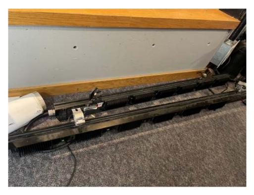
**Recommendation:** Dimming system wiring should be replaced with adequate circuits designed for an LED system. Relay racks should be supplied to allow for LED fixtures to be turned off when not in use, conserving electricity. Power distribution should be redesigned, replaced, and configured for efficient use to minimize extraneous cabling as much as possible, facilitating and speeding up deployment of new lighting plots.
