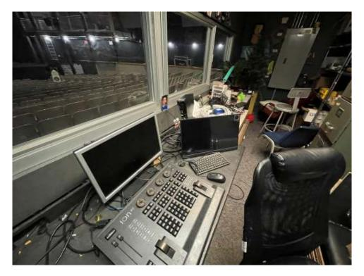
DMX distribution is outdated and not designed for the needs of a modern LED lighting system. Existing DMX outlets depend on jumping through to the next outlet to complete the run, making troubleshooting difficult.
