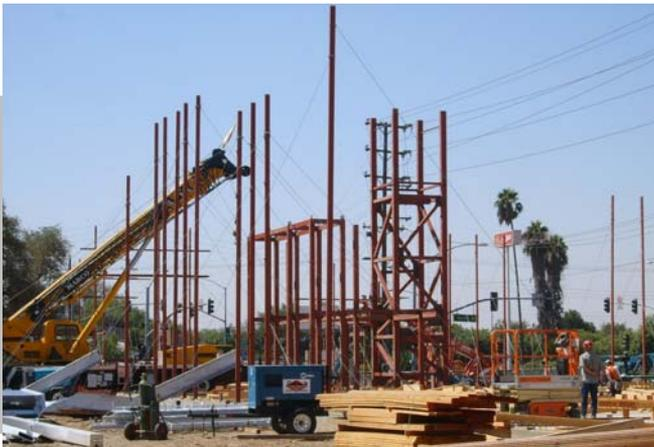
August 2011—project goes vertical with placement of structural steel for stair/elevator tower
