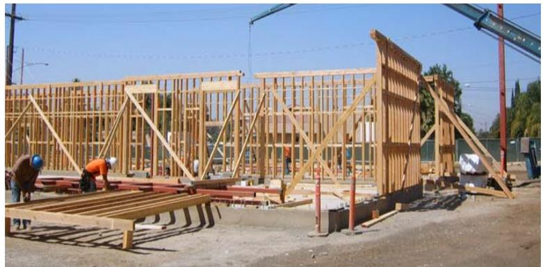
September 2011—With concrete foundation slab poured and cured, rough framing of first floor science building is underway
