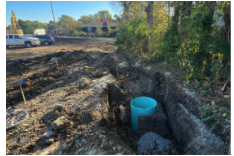
RHS: Installation of storm structure
