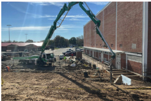
RSBS: Placement of concrete footings for PAC
