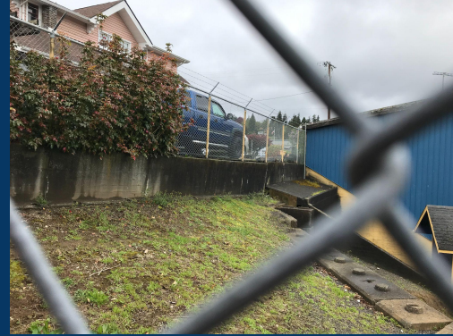
Stewart Field Retaining Wall
