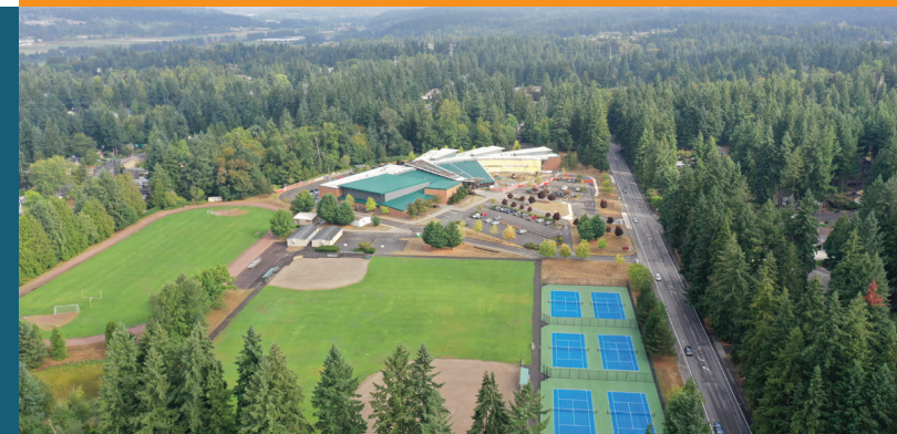
Upgraded Redmond Middle School tennis courts
