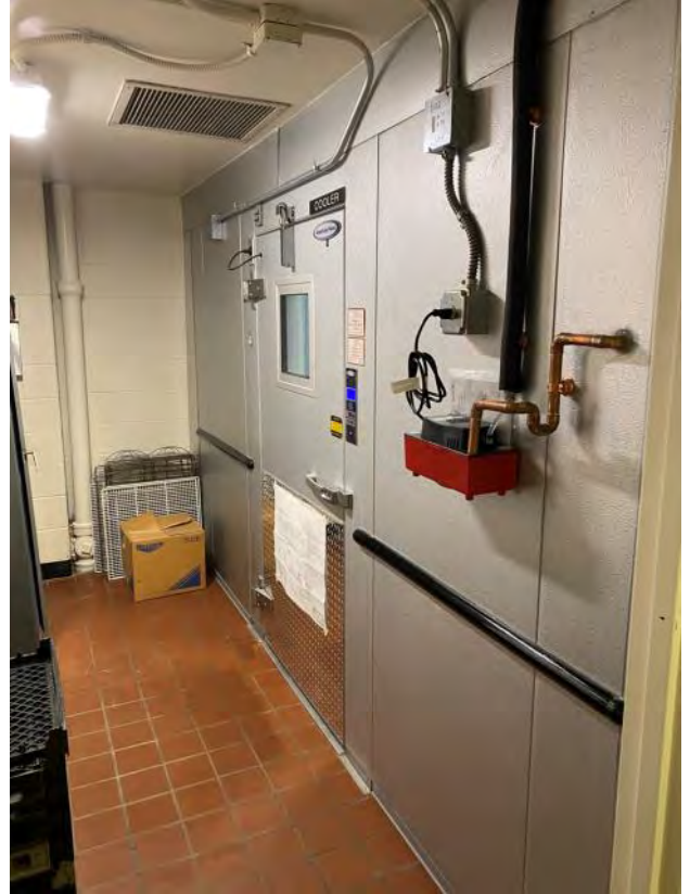
Scarlett Middle School Walk In Cooler Replacement
