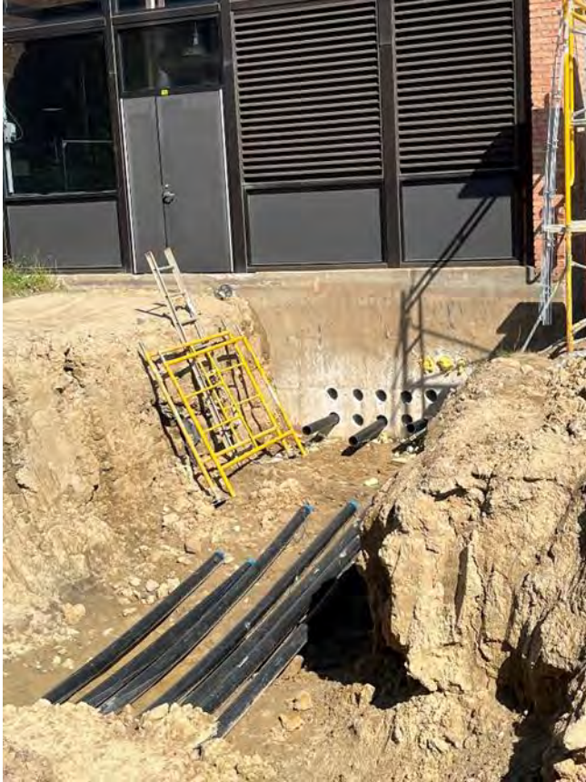
Geothermal piping installation
