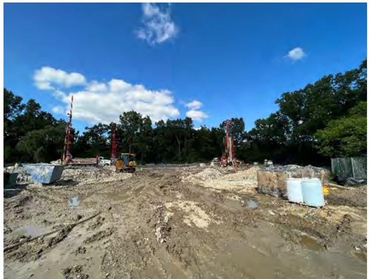
Drilling for Geothermal Pipe Installation
