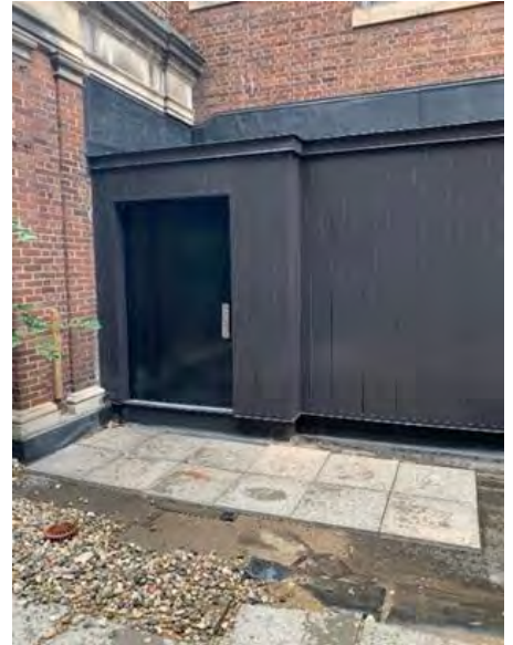
New Mechanical Room Entrance
