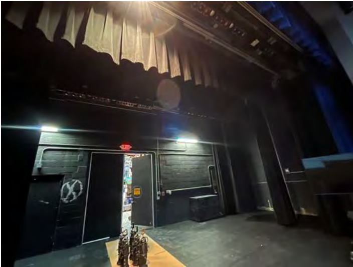
Pioneer Little Theater – Theater Rigging Replacement
