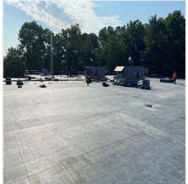
Bryant Elementary School – Roofing Improvements
