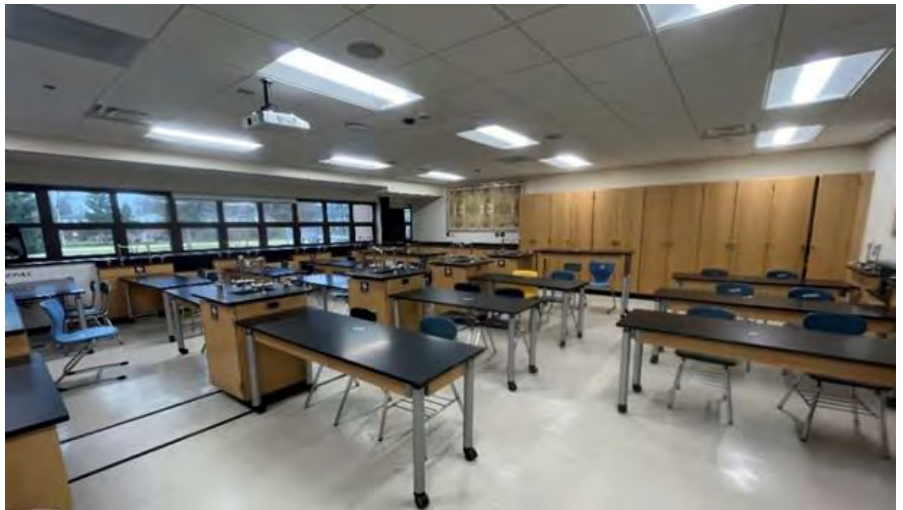
Air Conditioning, LED Lighting, and Ceiling Replacement
