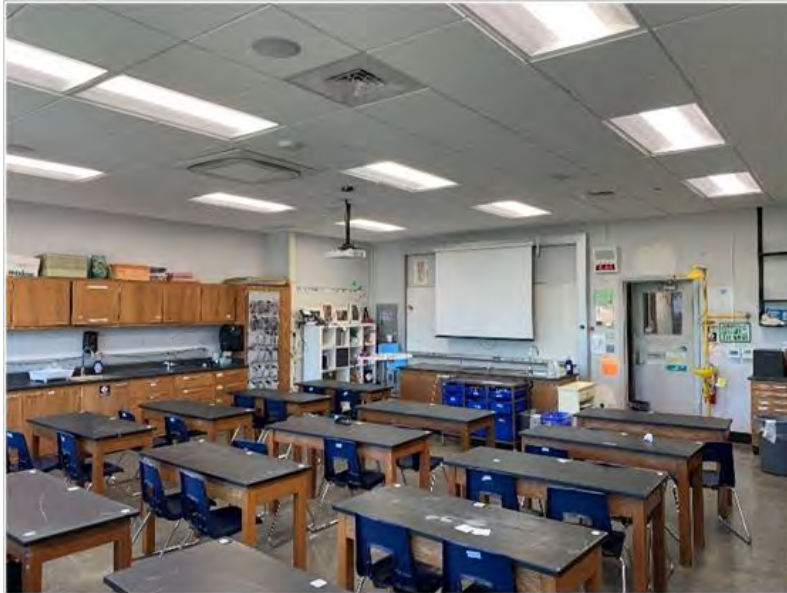
Air Conditioning, LED Lighting, and Ceiling Replacement
