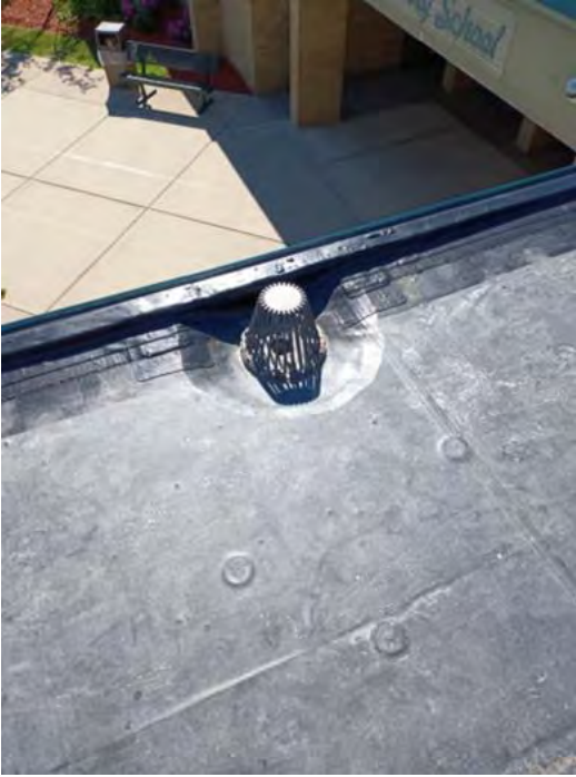
Mitchell Elementary – Roofing Improvements
