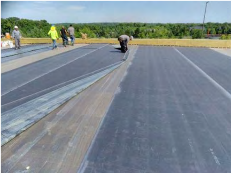
Huron High School – Roofing Improvements
