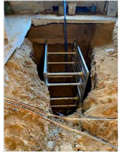
Carpenter Elementary School Storm Water Repair
