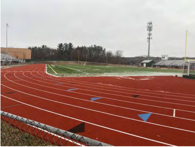
Huron High School Athletic Track Improvements
