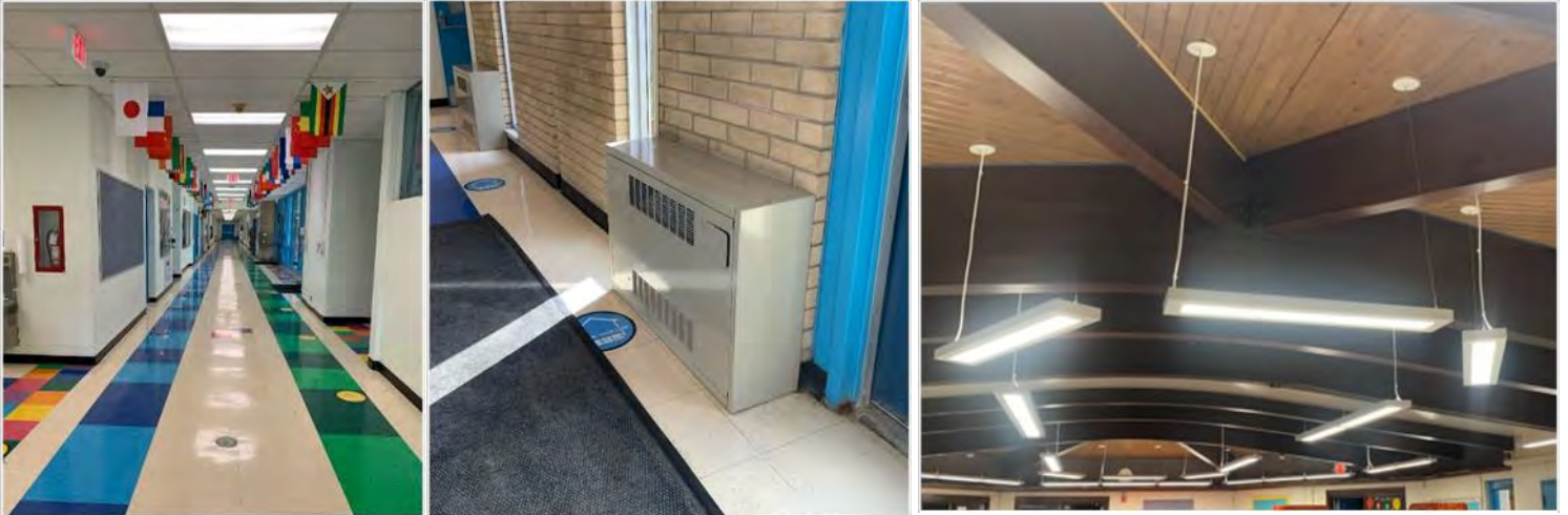
Lakewood Elementary School – Air Conditioning, LED Lighting, and Ceiling Replacement
