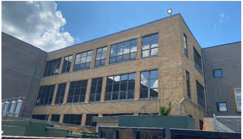
Masonry Restoration at Parapet & Stone Roof Coping
