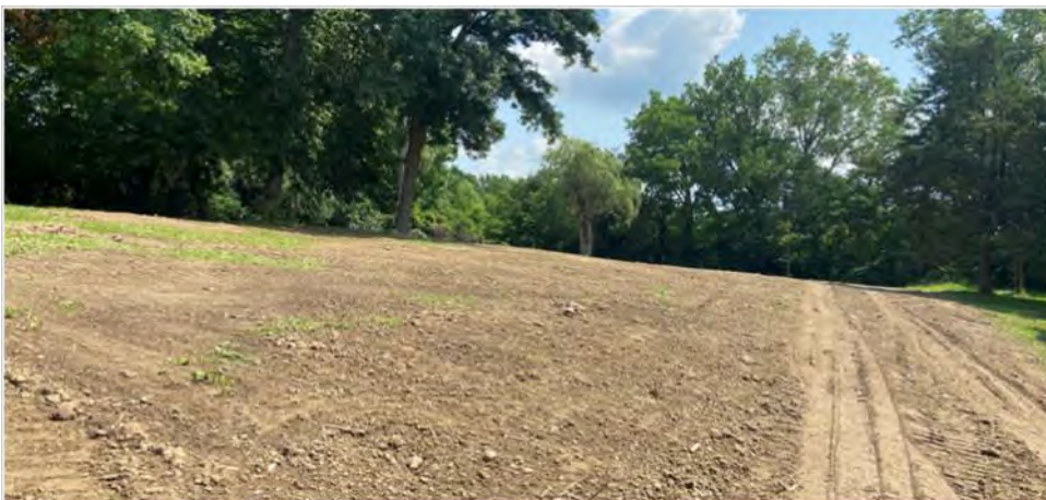
Nixon Road Structure Demolition
