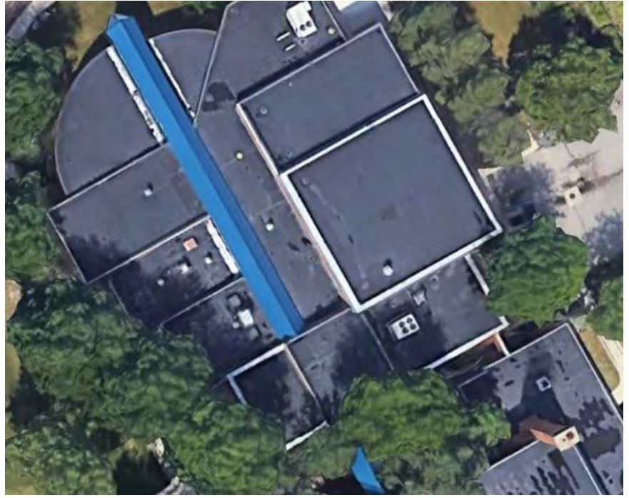
Pattengill Elementary – Roofing Improvements
