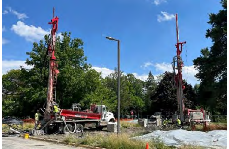
Drilling and installation of Geothermal Piping
