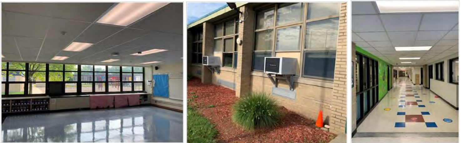
Mitchell Elementary School – Air Conditioning, LED Lighting, and Ceiling Replacement
