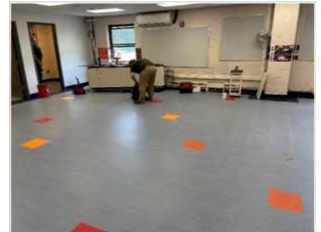
Carpenter Elementary School Storm Water Repair
