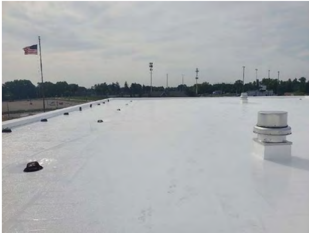
Pioneer High School – Roofing Improvements
