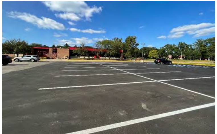
Parking Lot Replacement at Geothermal
