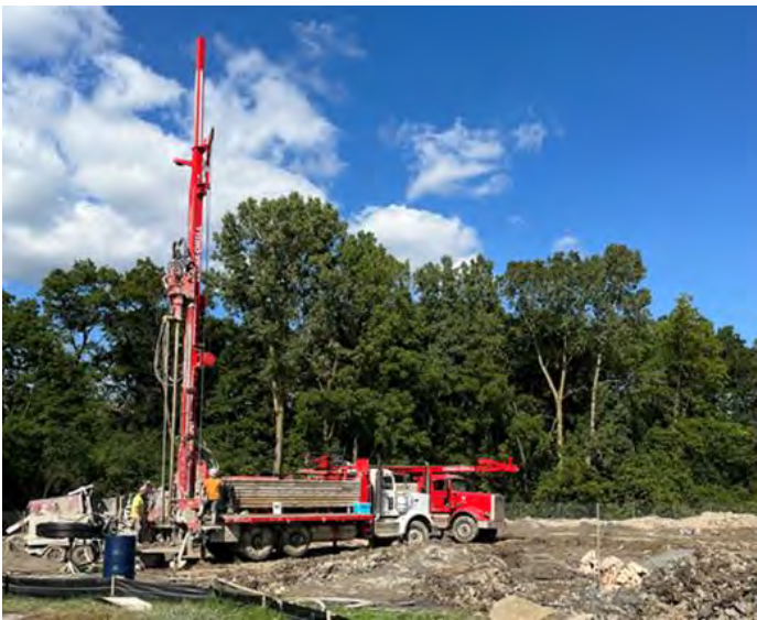
Drilling for Geothermal Pipe Installation
