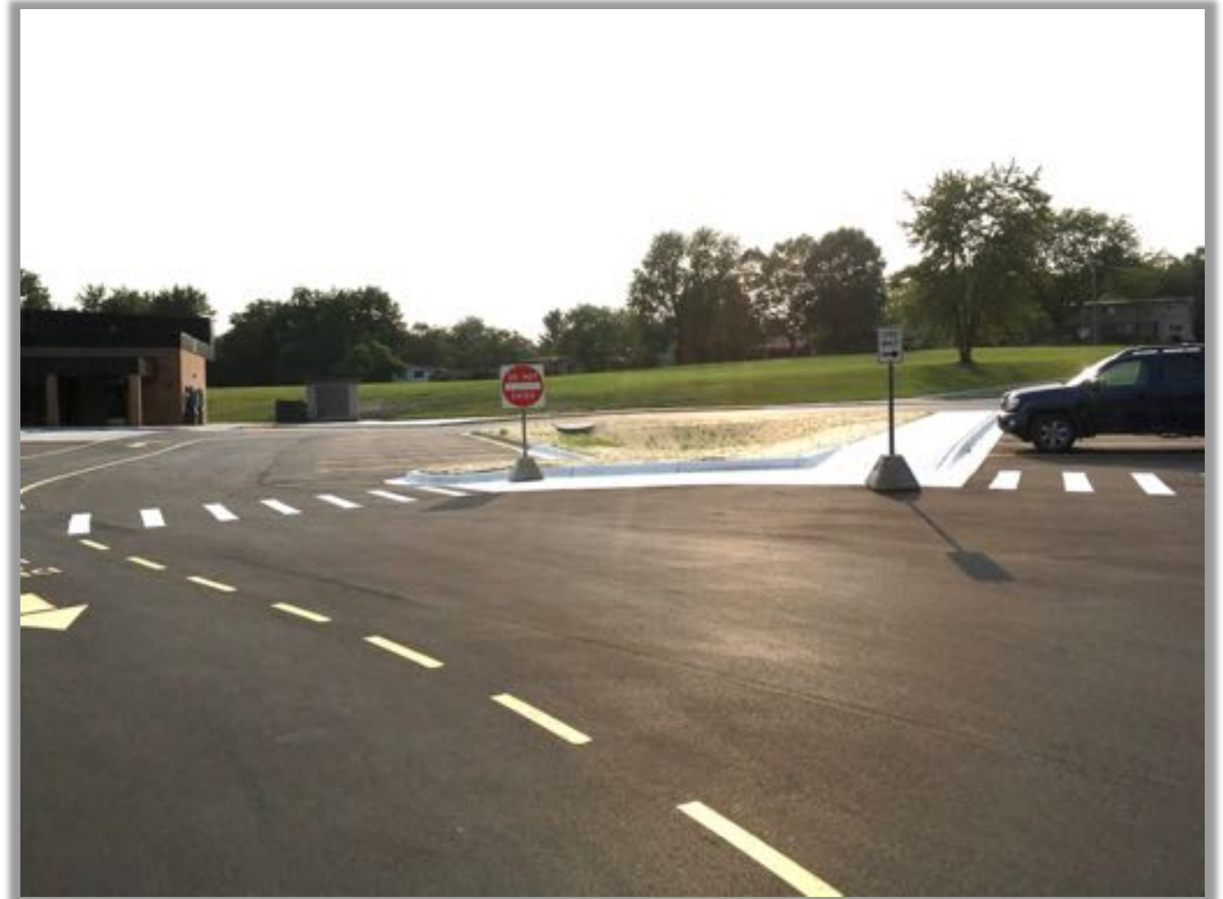
Allen ES site improvements
