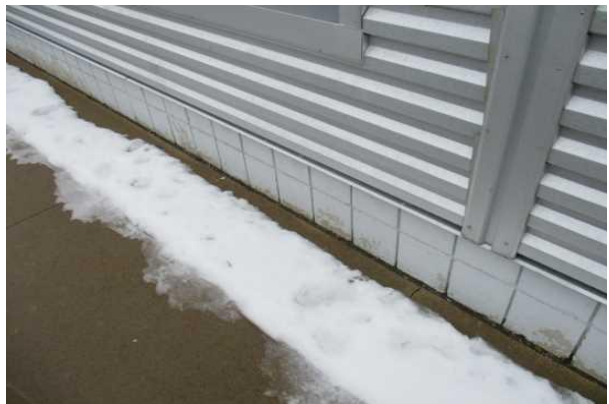
#18: EXTERIOR WALL PAINTED CMU
