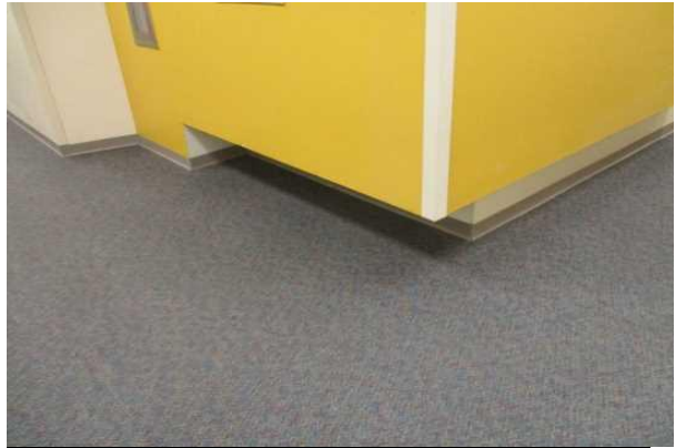
#8: INTERIOR WALLS AND CARPET
