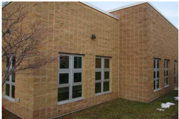
#10: CMU WALL AND WINDOWS
