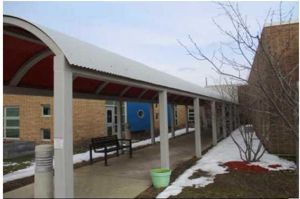
#20: ROOF, METAL AND BOLLARD LIGHTS
