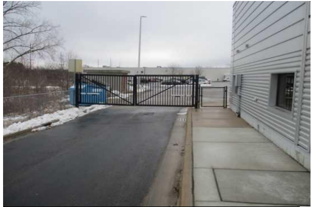
#62: SWING GATES WITH ELECTRIC OPENER
