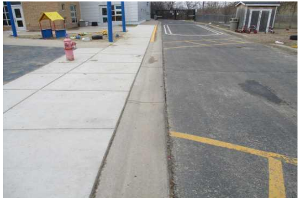
#64: REPLACED SIDEWALK, CONCRETE
