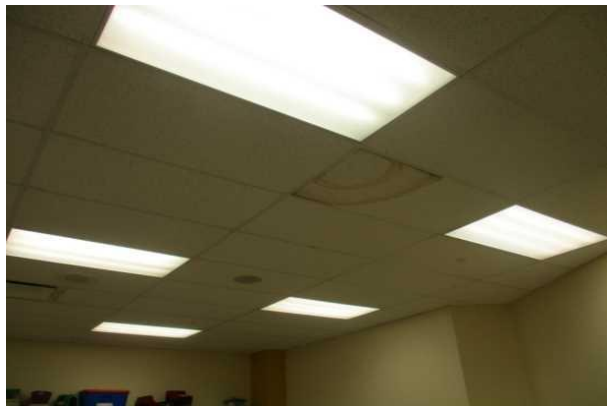
#22: INTERIOR CEILING FINISH
