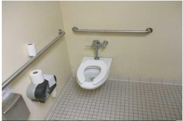
#32: GYPSUM BOARD REPAIR
