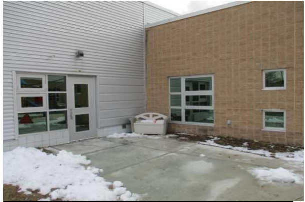
#14: CMU, SIDING AND WINDOWS
