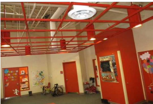
#23: PAINTED CEILING GRID
