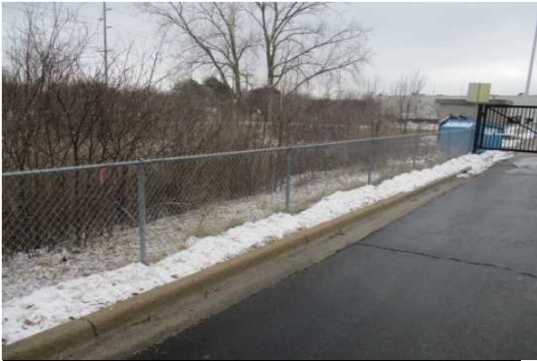
#61: CHAIN LINK FENCE
