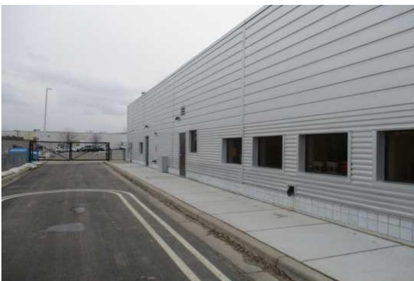
#11: METAL SIDING AND WINDOWS
