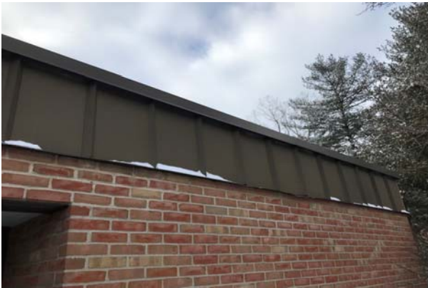
#9: EXTERIOR WALL, ALUMINUM SIDING
