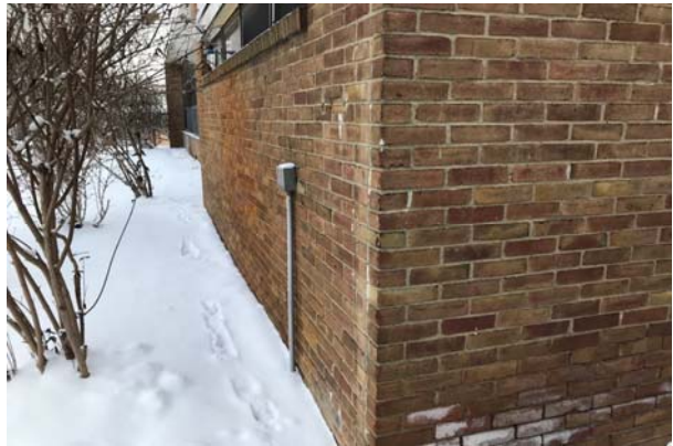
#10: EXTERIOR WALL, BRICK
