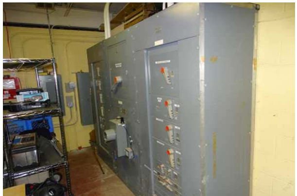
#42: BUILDING/MAIN SWITCHBOARD
