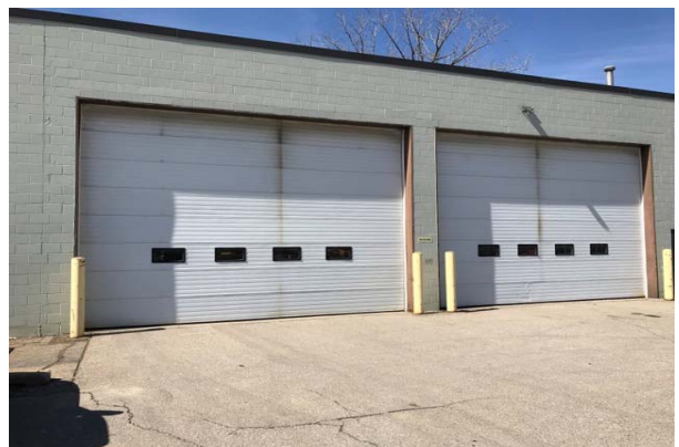
#12: OUTSIDE LOADING DOCK WITH OVERHEAD DOORS
