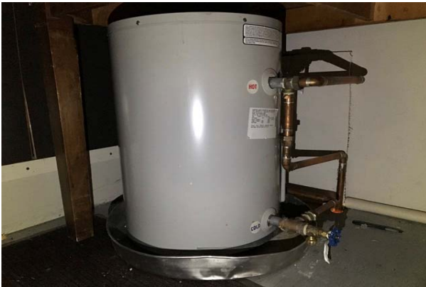
#21: TYPICAL DOMESTIC WATER HEATER
