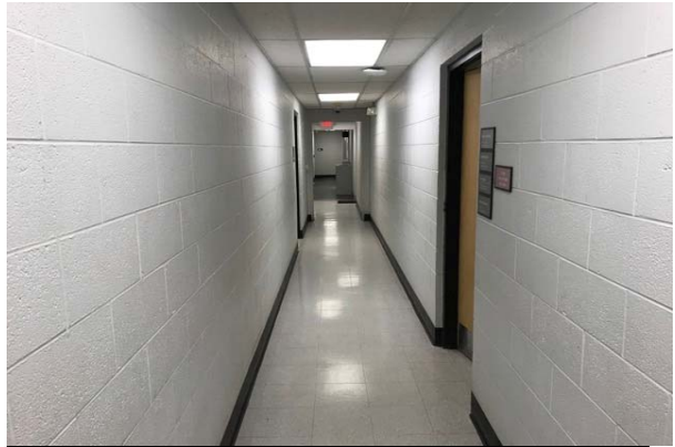
#14: LOWER LEVEL HALLWAY
