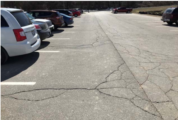
#33: TYPICAL PARKING LOT ASPHALT PAVING
