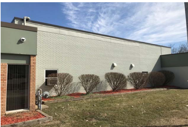
#11: TYPICAL EXTERIOR FACADE
