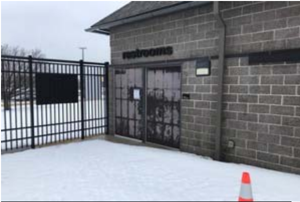
#31: EXTERIOR STEEL DOOR
