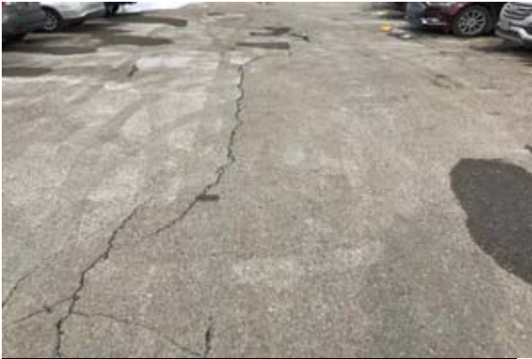
#7: ASPHALT PARKING LOT
