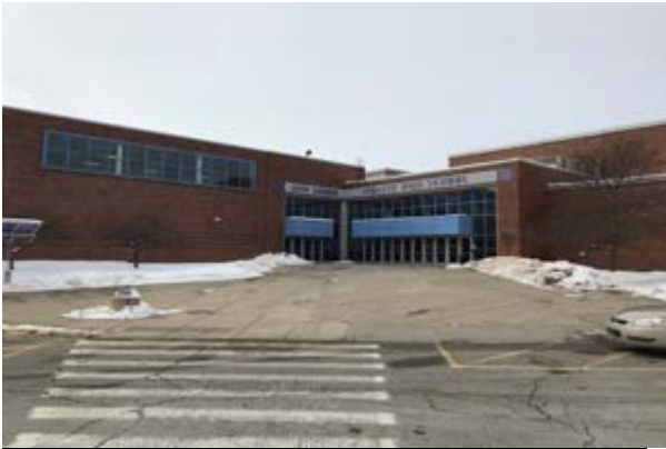
#1: FRONT MAIN ENTRANCE
