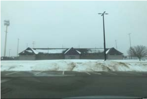
#19: EXTERIOR POLE LIGHTING
