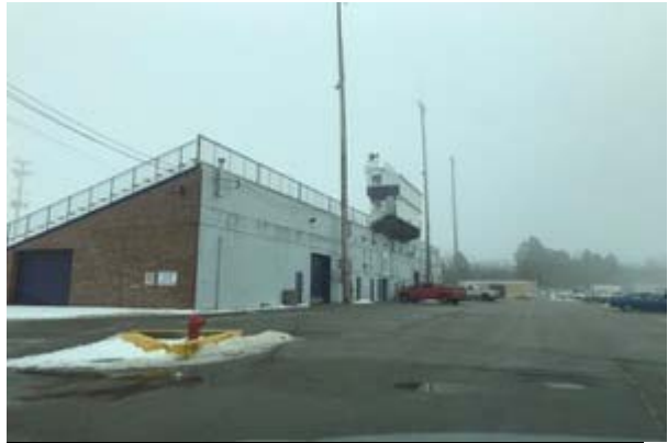
#20: STADIUM MAINTENANCE BUILDING
