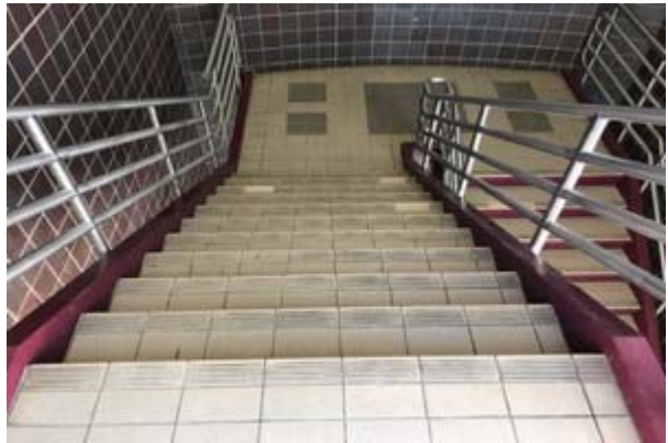
#28: QUARRY TILE STAIRS
