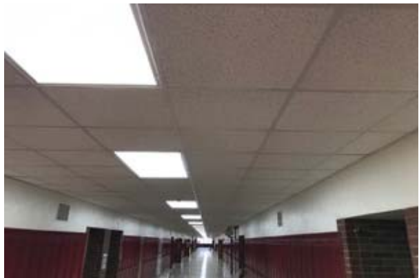
#72: SUSPENDED ACOUSTICAL TILE (ACT) CEILING
