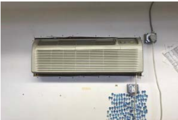
#41: HEAT/ COOLING MAINTENANCE BUILDING
