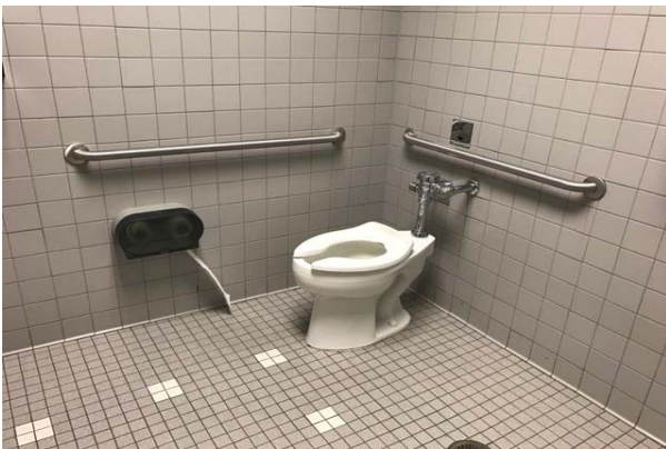
#29: TOILET, TANKLESS (WATER CLOSET)
