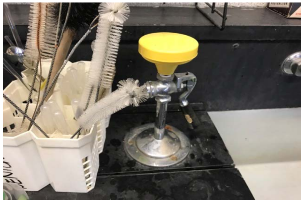
#24: EYE WASH STATION
