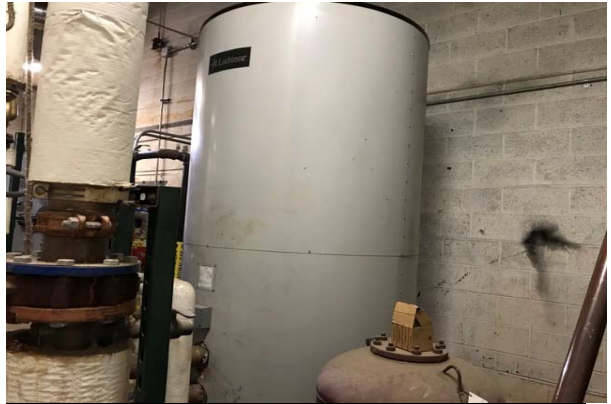
#32: WATER STORAGE TANK
