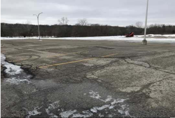
#7: ASPHALT PARKING LOT
