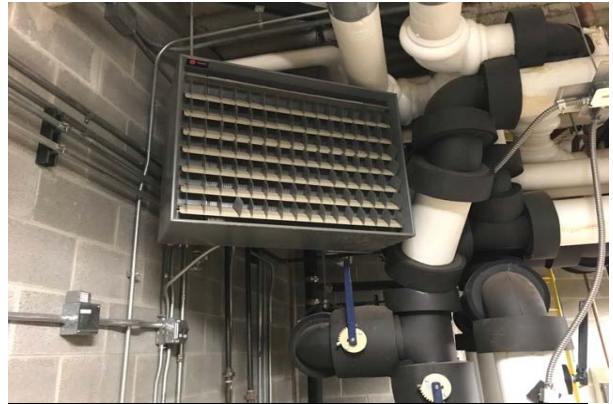
#44: UNIT HEATER, HYDRONIC
