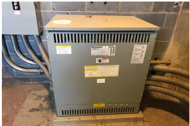
#54: SECONDARY TRANSFORMER
