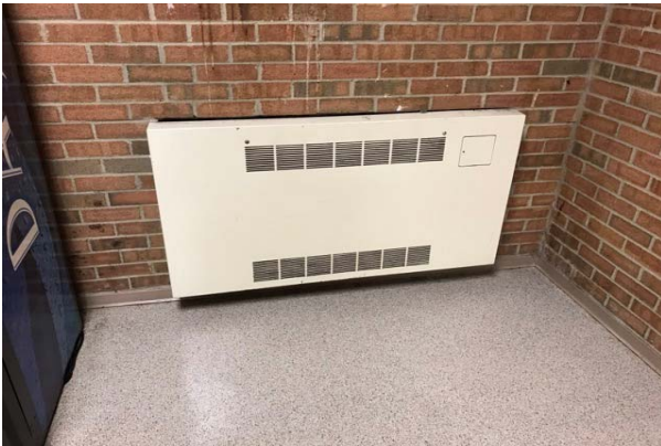
#39: CABINET HEATER, ELECTRIC
