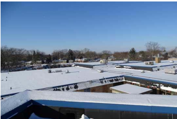
#17: ROOF, SINGLE-PLY EPDM MEMBRANE
