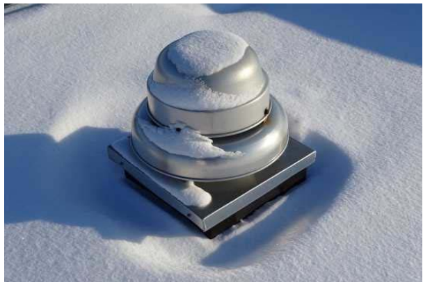
#34: EXHAUST FAN, CENTRIFUGAL,
