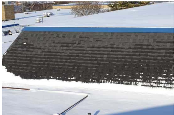
#18: ROOF, ASPHALT SHINGLE
