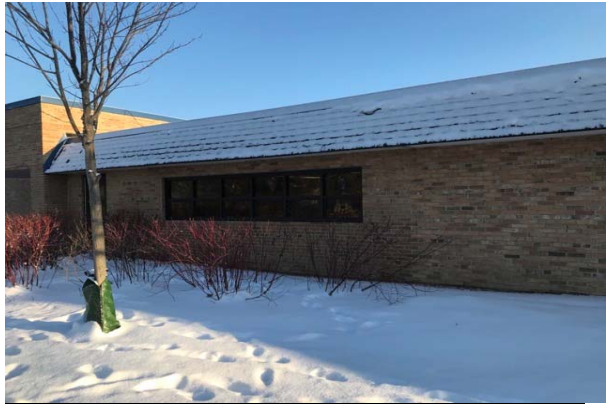
#20: EXTERIOR WALL, BRICK
