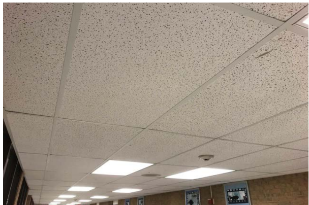
#48: INTERIOR CEILING SUSPENDED ACOUSTICAL TILE (ACT)
