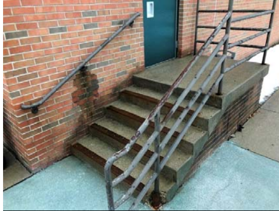
PHOTO #12: CONCRETE STAIRS
