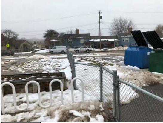
PHOTO #11: CHAIN LINK PERIMETER FENCING
