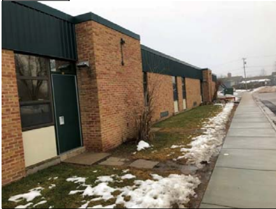
PHOTO #3: EAST ELEVATION
