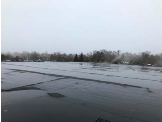
PHOTO #13: SINGLE-PLY ROOFING
