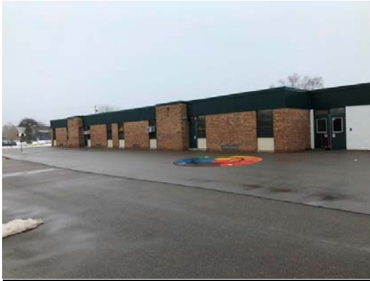
PHOTO #1: WEST ELEVATION
