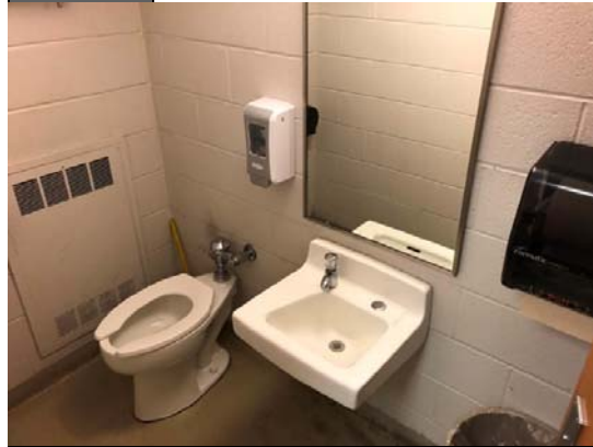
PHOTO #34: CLASSROOM RESTROOM
