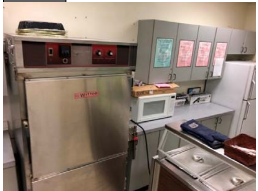
PHOTO #24: KITCHEN EQUIPMENT
