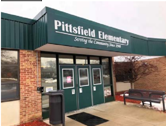
PHOTO #5: MAIN ENTRANCE DOORS
