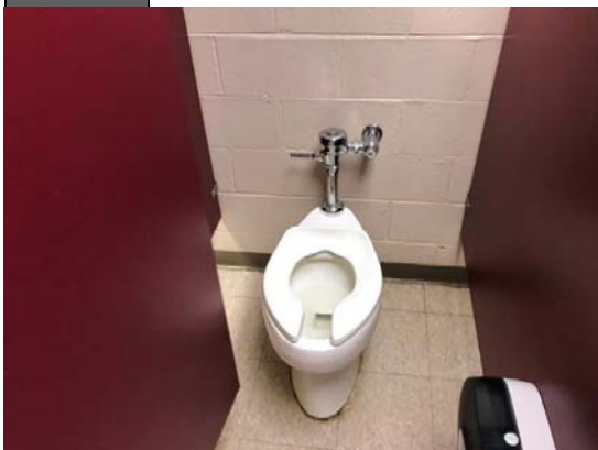
PHOTO #35: RESTROOM STALL
