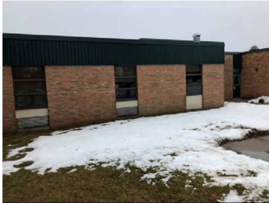
PHOTO #2: NORTH ELEVATION
