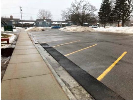
PHOTO #7: CONCRETE SIDEWALKS AND ASPHALT PAVEMENT
