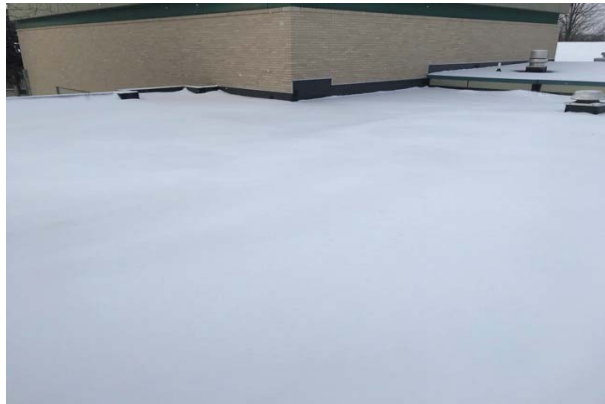
#28: ROOF, BUILT-UP MEMBRANE
