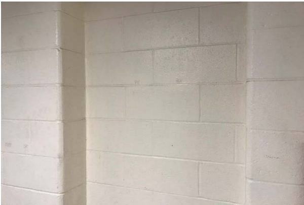
#27: STRUCTURAL WALLS, CMU
