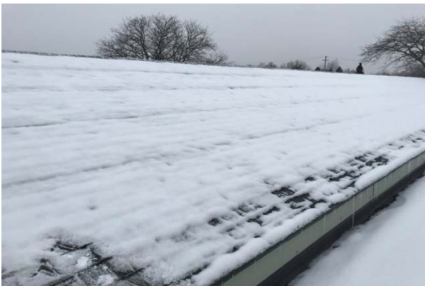
#29: ROOF, ASPHALT SHINGLE
