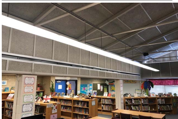
#12: SUSPENDED ACOUSTICAL TILE
