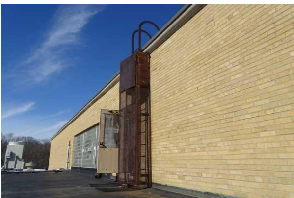
#23: ROOF ACCESS LADDER
