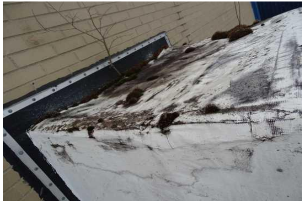
#46: HVAC SYSTEM DUCTWORK GROWTH
