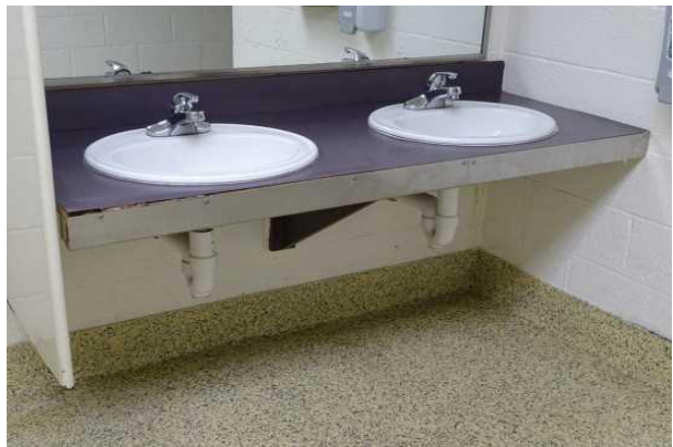
#28: REST ROOM COUNTER AND SINKS
