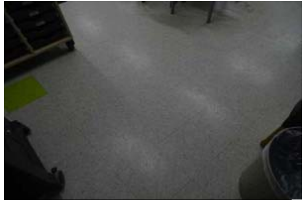
#14: SOUTH ANCILLARY STRUCTURE, VINYL TILE
