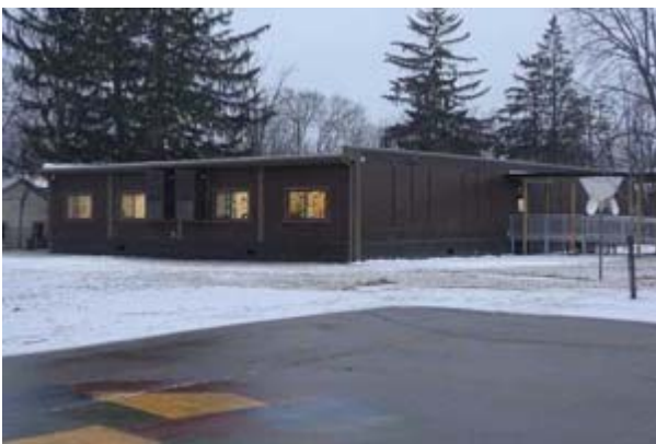
#11: SOUTH ANCILLARY STRUCTURE, VINYL SIDING
