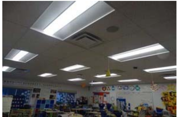
#16: SOUTH ANCILLARY STRUCTURE, SUSPENDED ACOUSTICAL TILE
