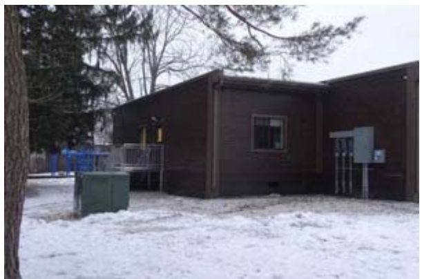
#6: SOUTH ANCILLARY STRUCTURE REAR ELEVATION
