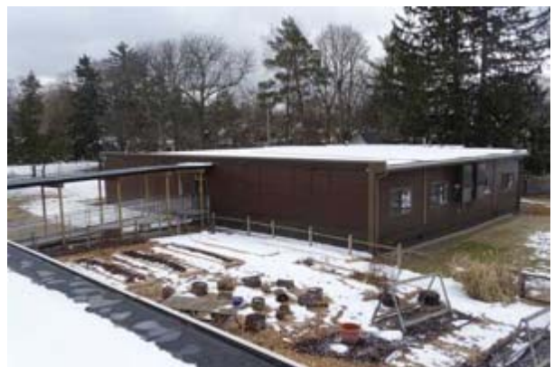
#12: SOUTH ANCILLARY STRUCTURE, ROOF
