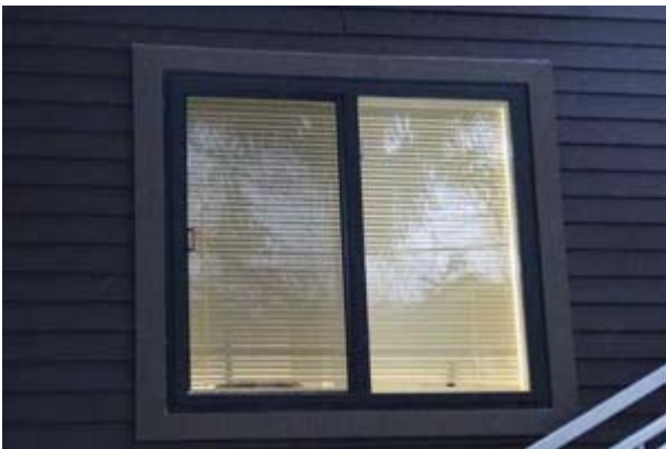
#17: SOUTH ANCILLARY STRUCTURE, WINDOWS
