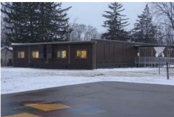
#5: SOUTH ANCILLARY STRUCTURE FRONT ELEVATION
