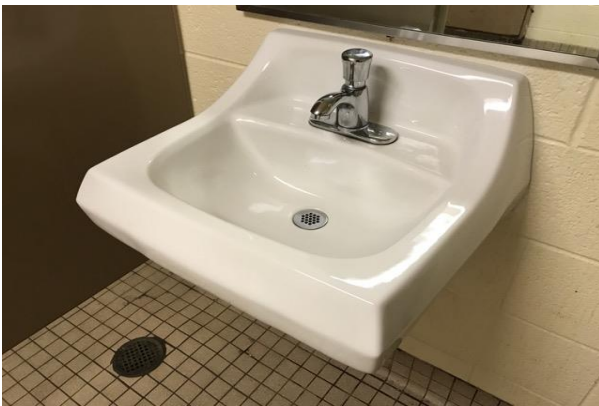
#39: SINK, VIRTUOUS CHINA, REPLACE
