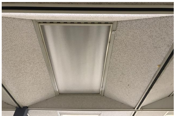
#42: SUSPENDED ACOUSTICAL CEILING TILE (ACT), REPLACE
