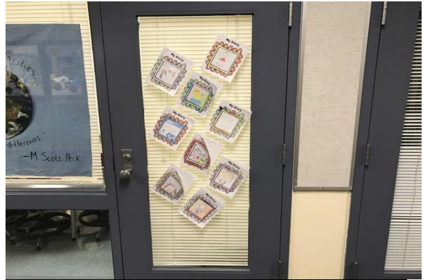
#44: INTERIOR DOOR, FULLY GLAZED, REPLACE
