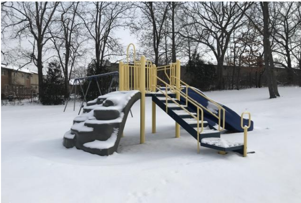
#15: PLAY STRUCTURE, REPLACE
