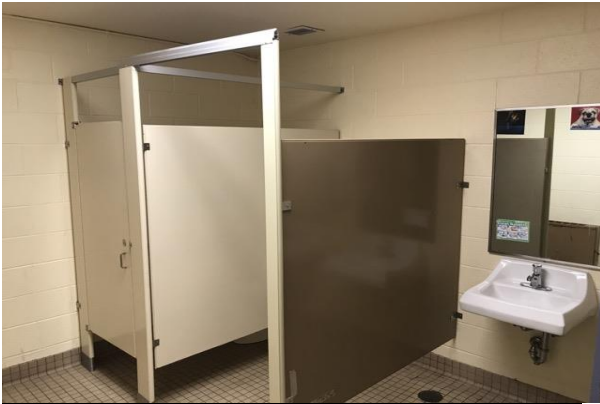
#31: TOILET PARTITIONS, METAL, REPLACE
