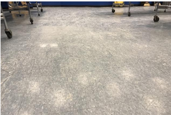
#11: VINYL CUT TILE (VCT), REPLACE
