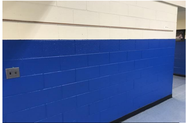
#14: CMU BLOCKS, PREP AND PAINT
