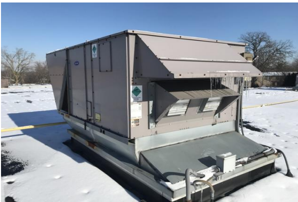
#27: PACKAGE UNIT, ROOFTOP, REPLACE
