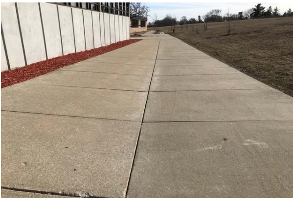
#51: TYPICAL CONCRETE SIDEWALK
