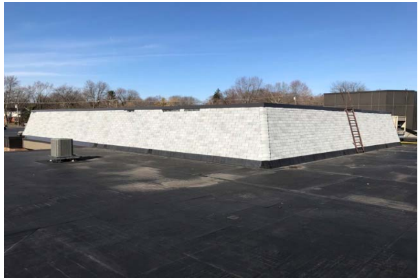
#10: MANSARD ROOF, ASPHALT SHINGLED
