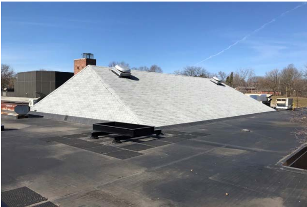
#9: HIP ROOF, ASPHALT SHINGLED
