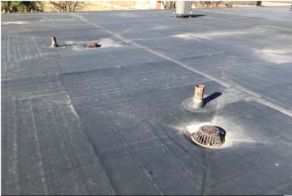
#7: FLAT ROOF, EPDM SINGLE-PLY
