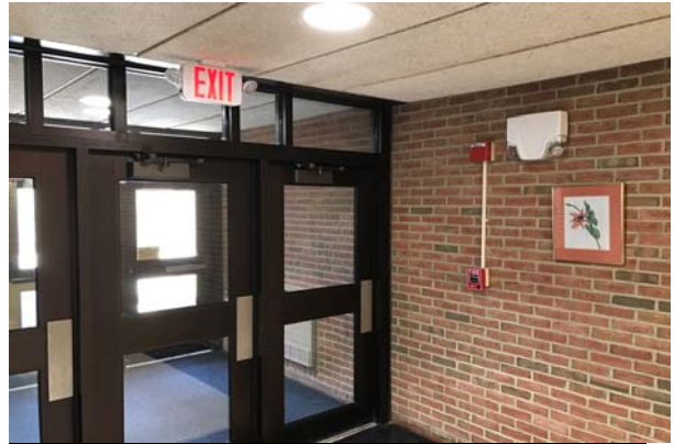
#44: TYPICAL FIRE ALARM COMPONENTS
