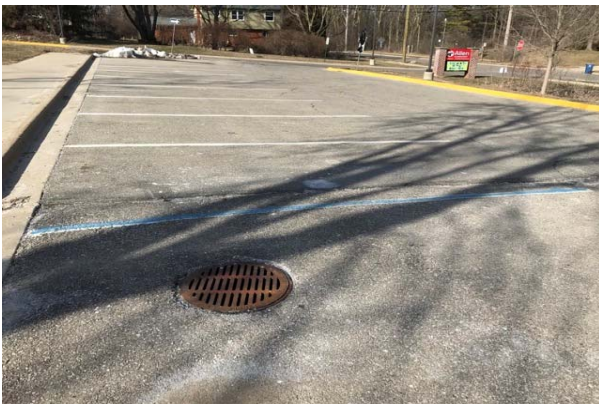
#47: FRONT ASPHALT PAVED PARKING LOT
