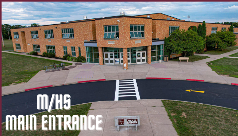
NORTH END (Hinsdale Drive)
