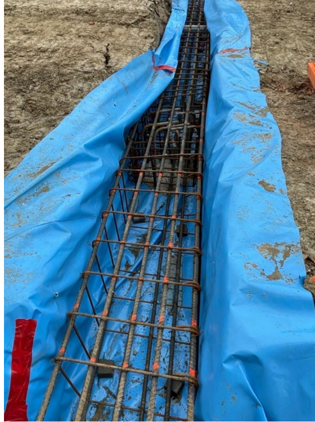
Item #04: Reinforcement steel size and spacing at grade at grade beam.
