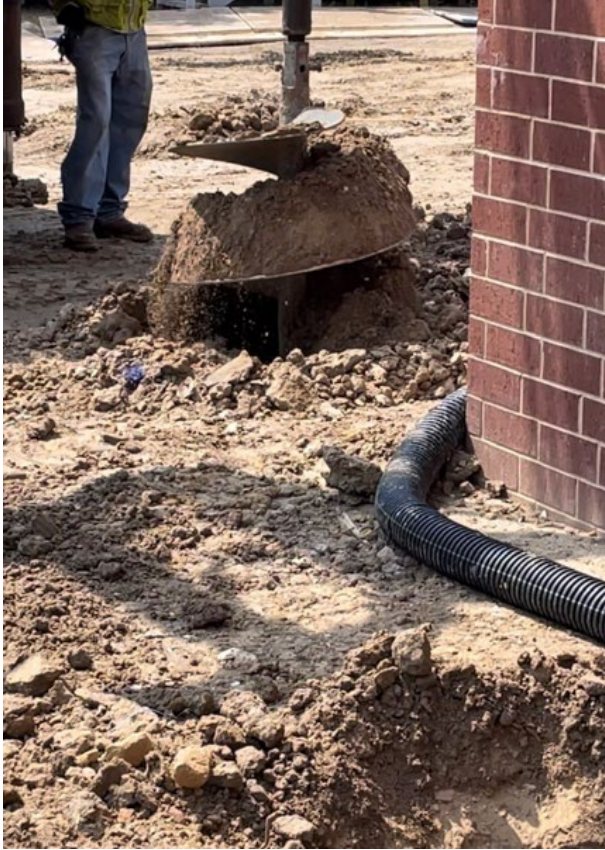
Item #03: Pier Drilling
