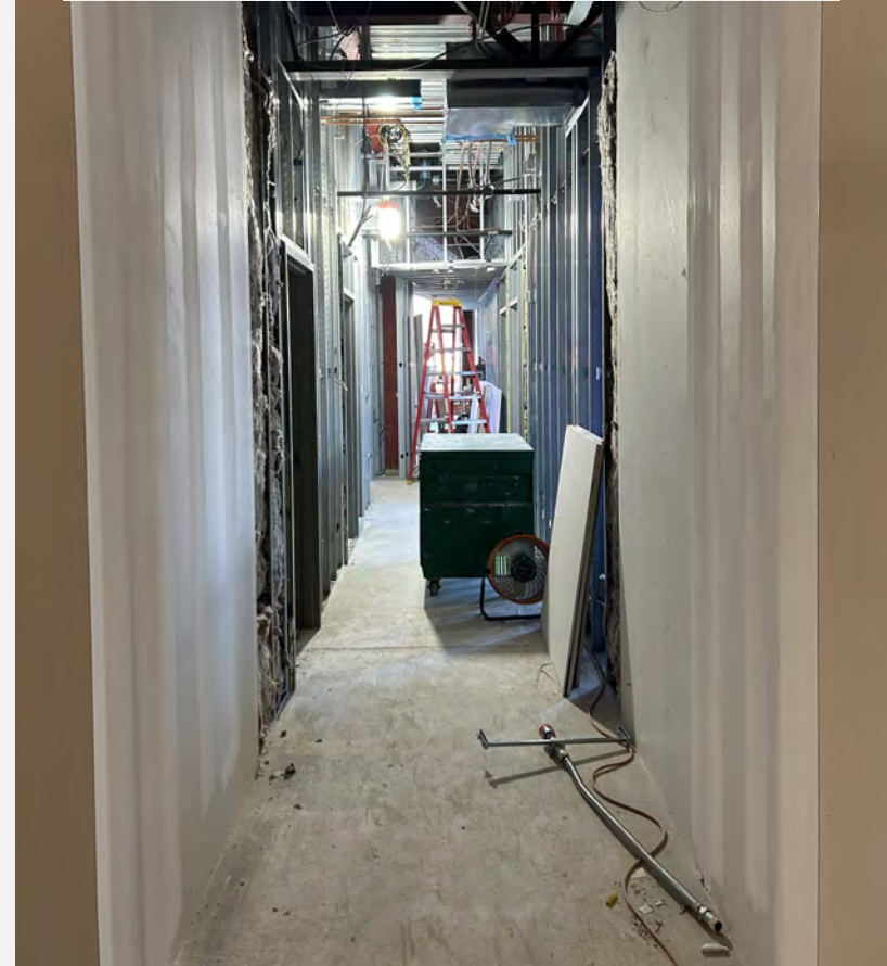
Hallway Leading to Principal Offices/Waiting Room
