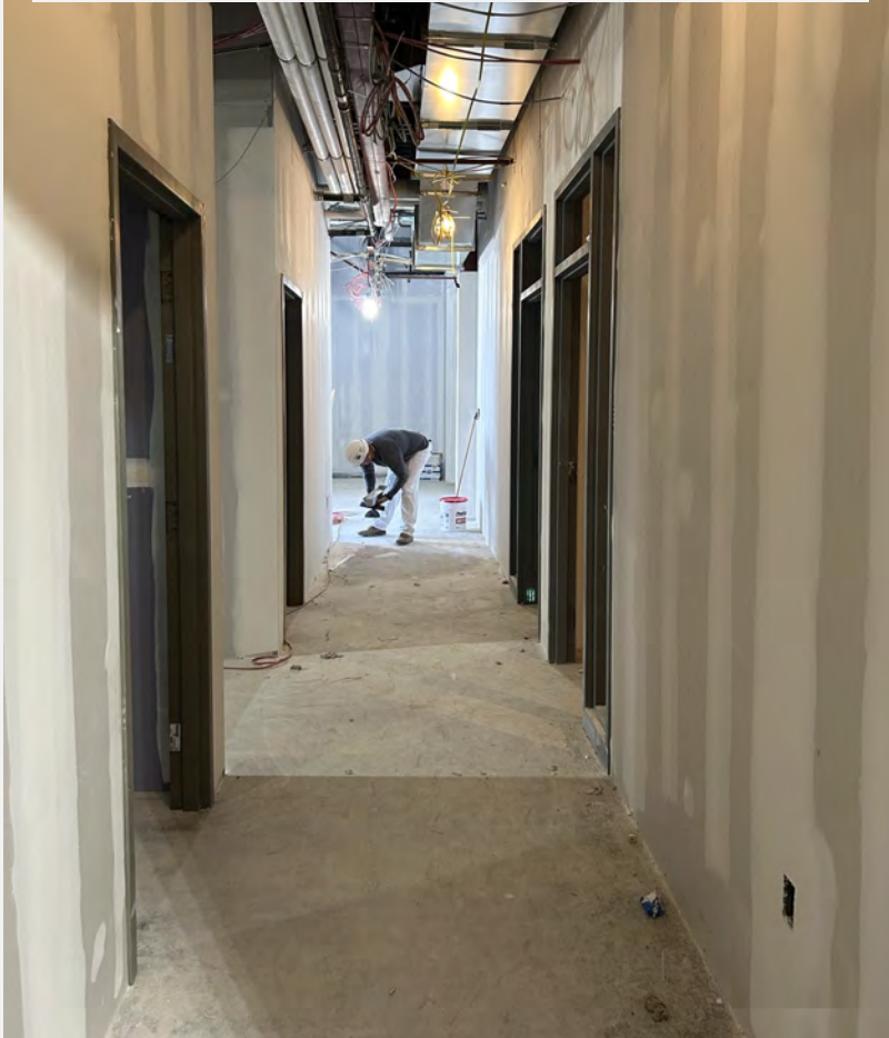
Hallway Leading to AD Office
