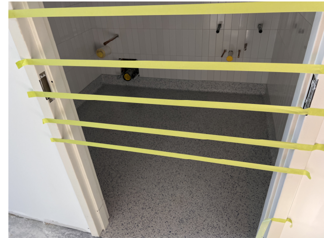
Epoxy Floor Complete
