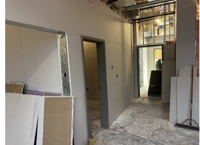
Back of House Drywall Begins
