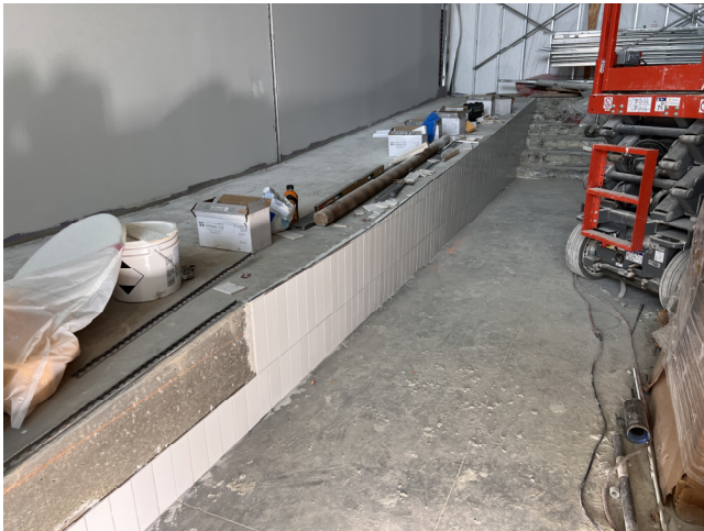
Lobby Finishes Ongoing
