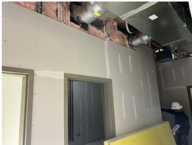
Drywall Tape & Finish
