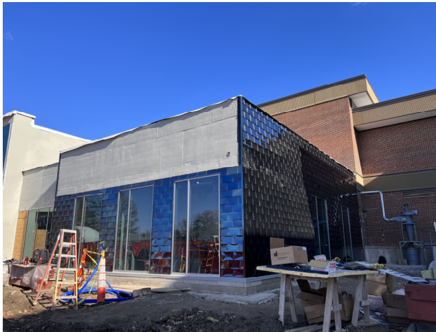
Exterior Metal Panel System
