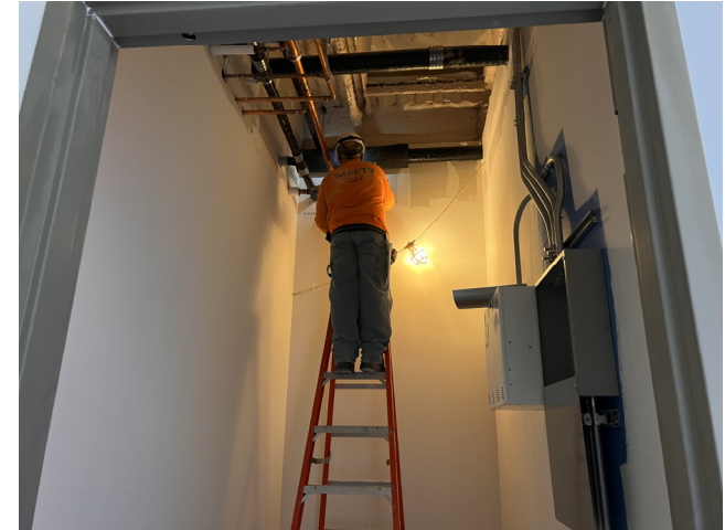
Insulating Overhead MEP
