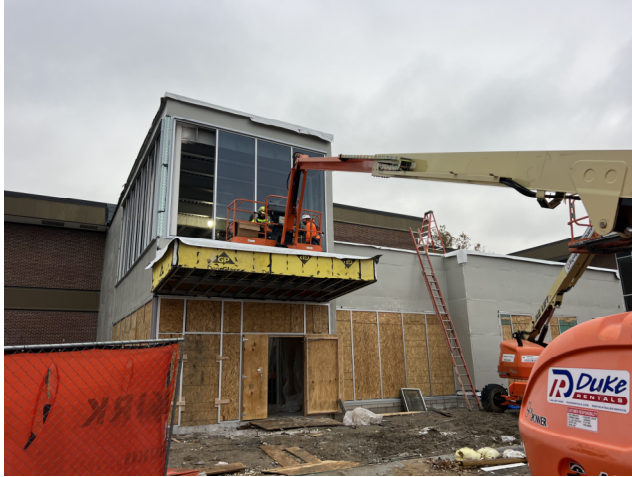
Glazing at New Entrance
