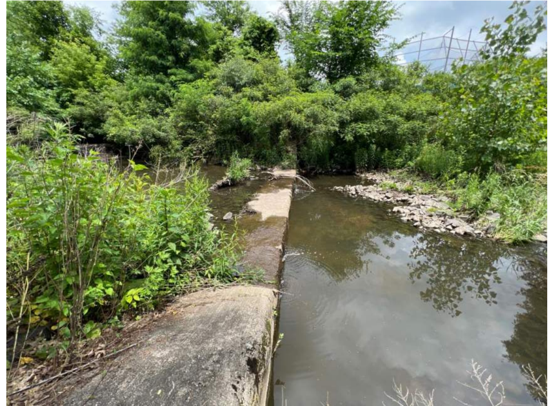
St. Joseph's Brook Concrete Weir
