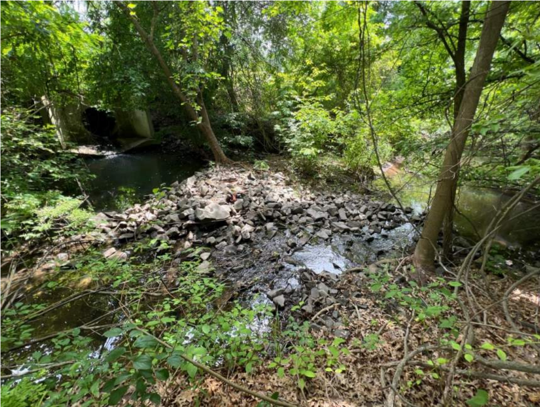
St. Joseph's Brook Armoring At Ball Field Culvert
