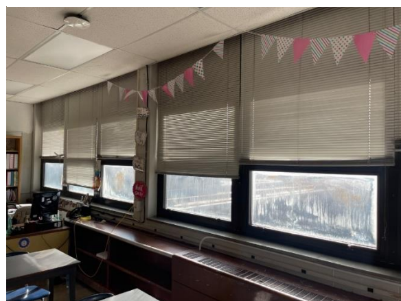
Typical windows with broken seals
