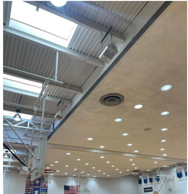
Gym soffit reported to contain asbestos
