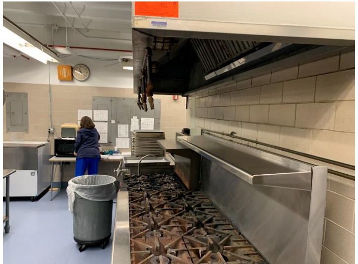
Non-conforming Type I kitchen hood
