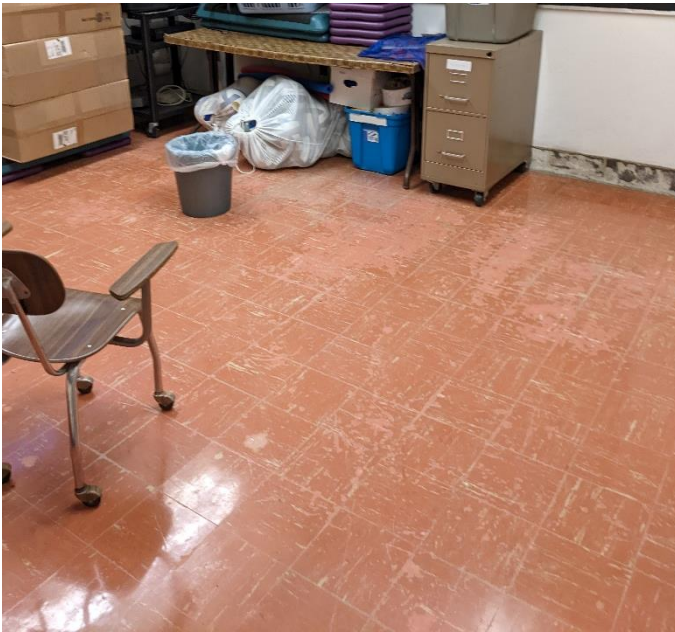
Asbestos floor tile
