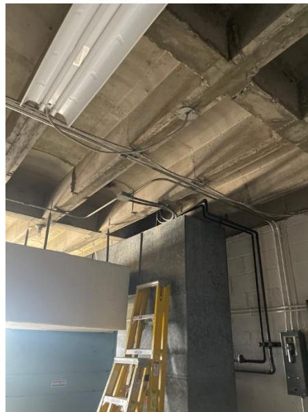
Precast concrete planks
