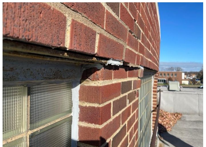
Shifting parapet over lintel
