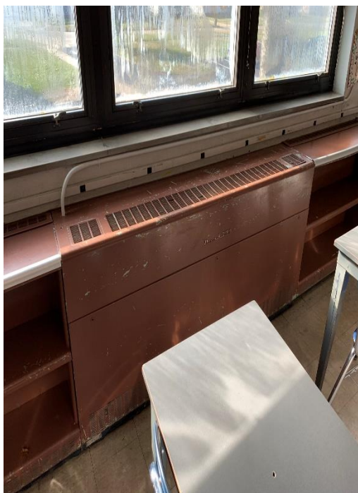
Unit Ventilator without AC
