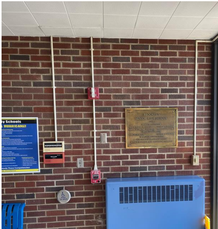
Manual fire alarm pull and strobe
