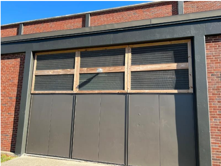
Exterior hollow metal doors
