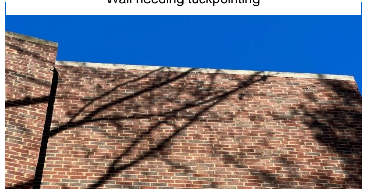
Parapet needing rebuilt
