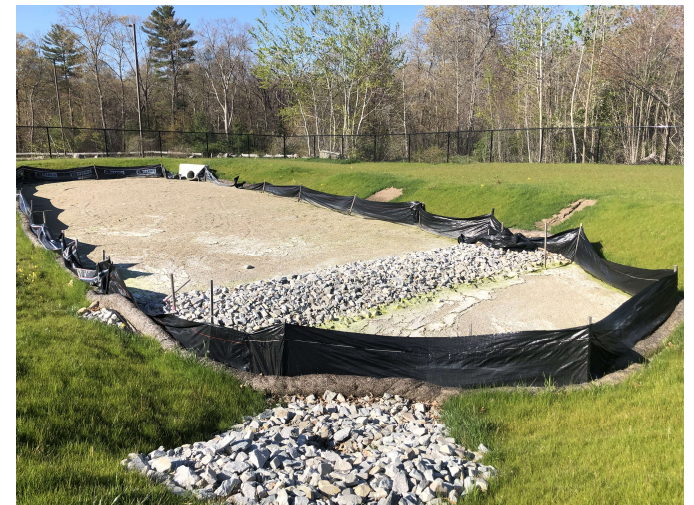
Sand Filter (construction photo)
