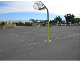
ed area. The existing pavement should be slurry sealed and restriped.
