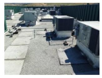
sealant around the exposed duct units have also begun to fail. The general roofing is in fair condition, however minor area of ponding water and granule loss is evident.
