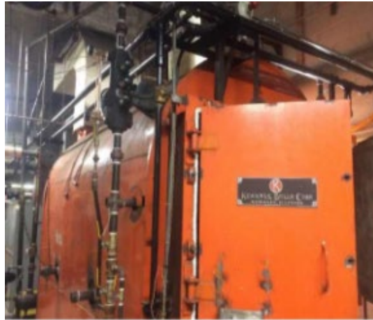
D3021 Boilers:- View of HW Boiler - Oil/Gas - 1010 to 4505 MBH (30 to 134 BHP)
