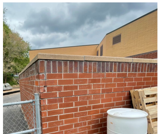
Brick walls require replacement
