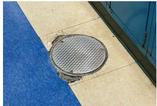
Movement of plumbing clean-outs
