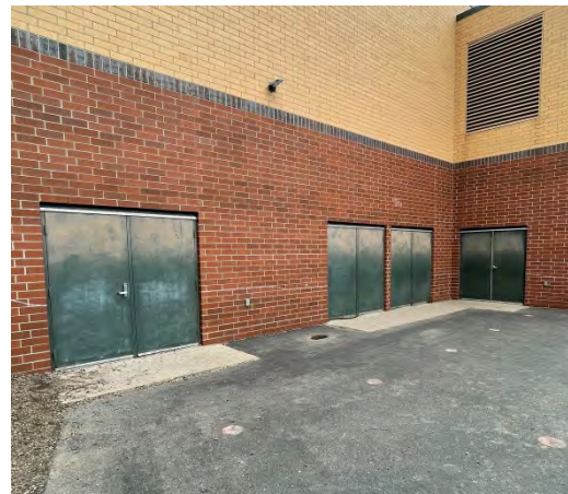
Hollow metal doors at gym and storage
