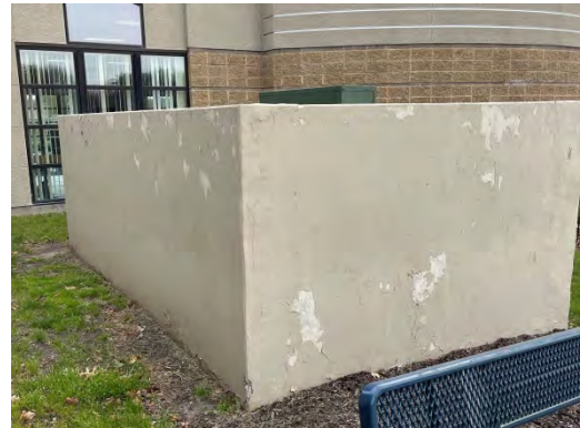
Stucco walls at transformer require repair
