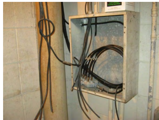
CATV system wiring
