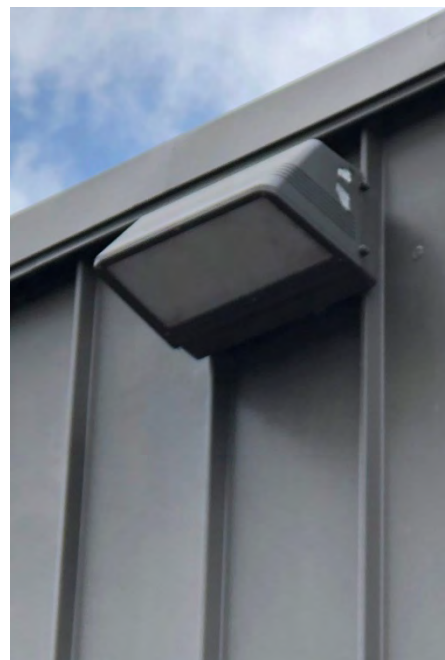
Exterior led lighting fixture
