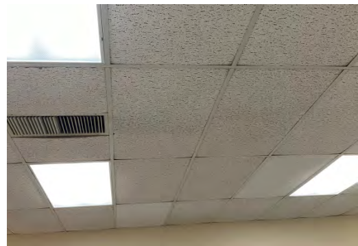
Acoustical tile sagging, typical
