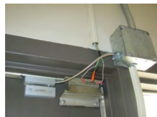
Security system contact switch
