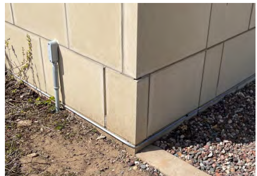
Mortar missing from manufactured stone
