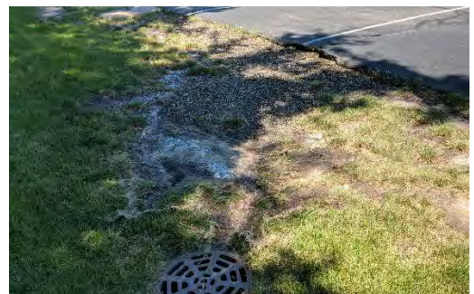
Erosion at upper play area – map grid J3-4
