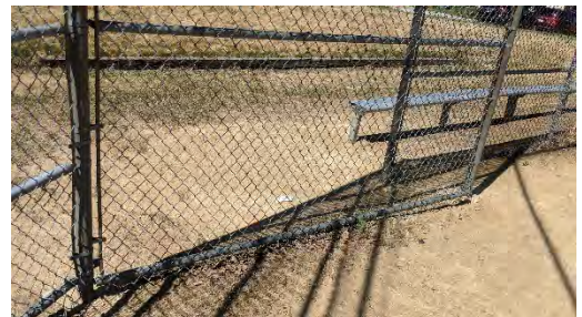
Repair backstop bottom rail – map grid H2
