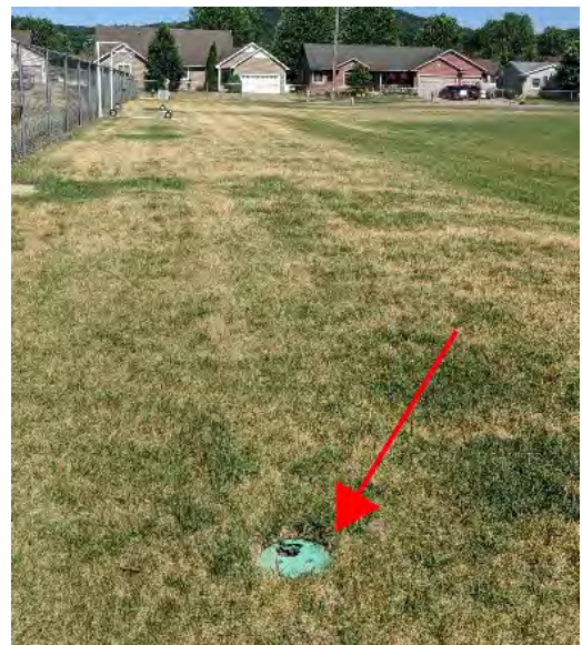
Broken valve box cover
