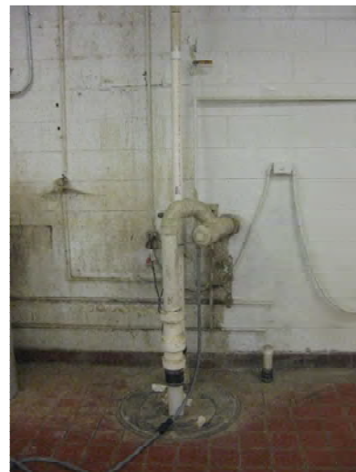
Sanitary sump and pump
