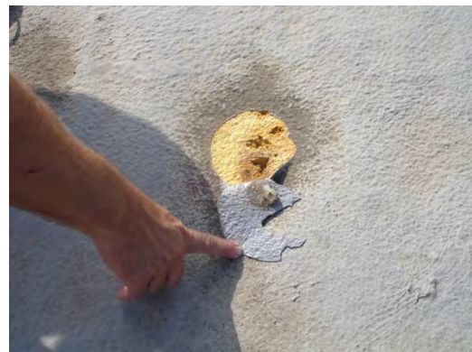
Example of holes created in foam causing deterioration
