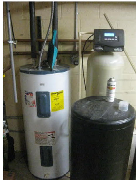
Water heater and softener
