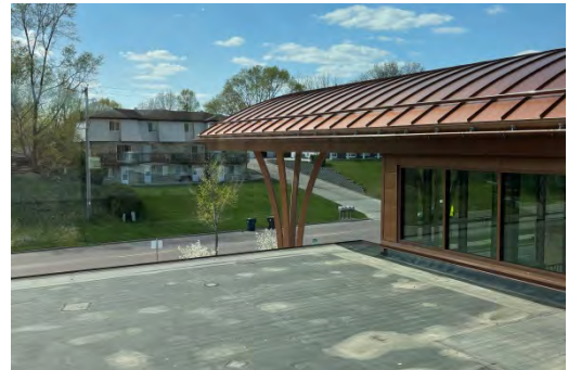
Fully adhered roof at 2014 additions.
