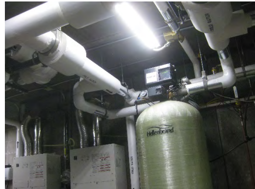
Water heaters and softener (8705)
