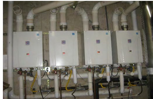
Water heaters and softener
