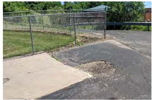
Pavement failure – map grid J3
