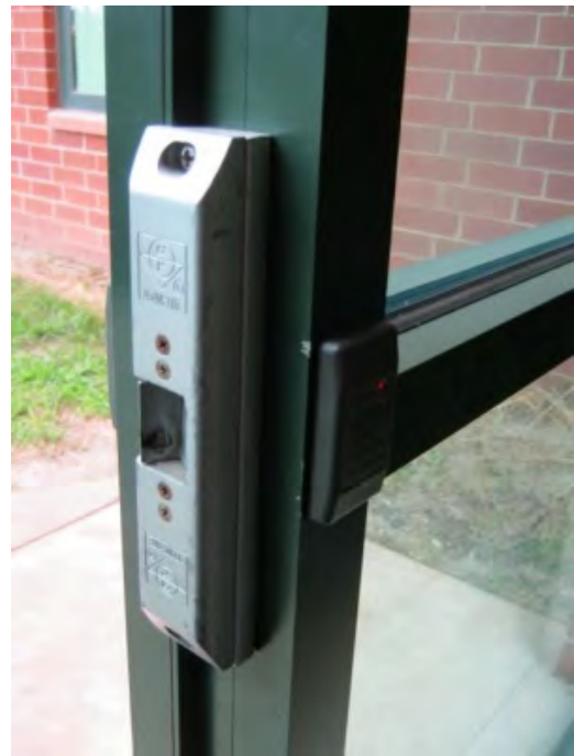
Electronic door access control system
