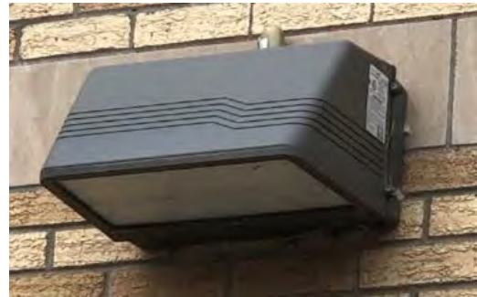
Exterior LED lighting fixtures
