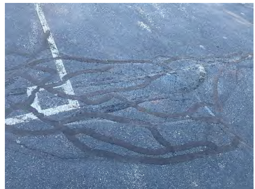
Areas of pavement failure (map grid D-E5 and D3)
