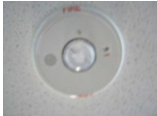
Fire alarm notification device
