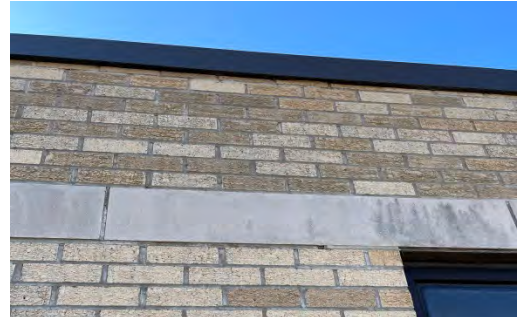
Tuck point and joint repair required at stone band above windows
