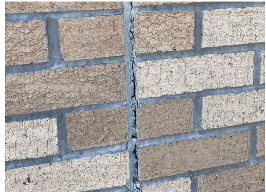
Multiple control joints demonstrate signs of aging and cracking
