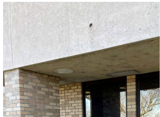
Multiple breakages in EIFS surface
