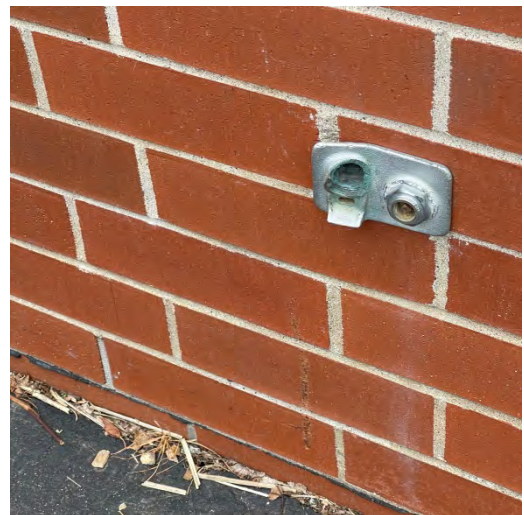
Damaged hose bib and membrane flashing deteriorated at base of wall
