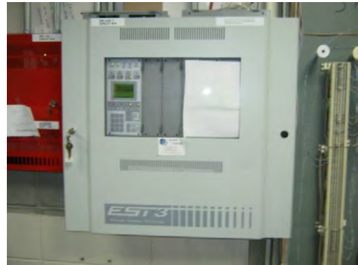
Fire alarm control panel
