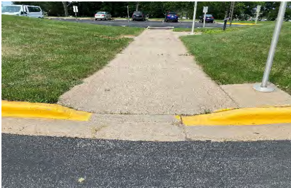
No detectable warning fields – map grid E4 and E5
