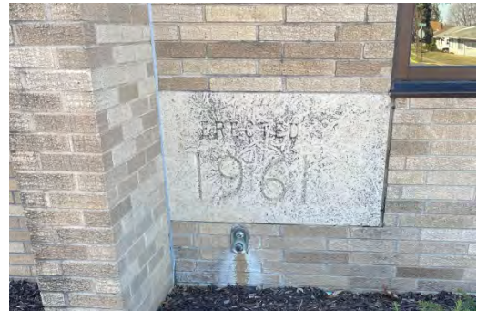
Sealant required at various hose bibs
