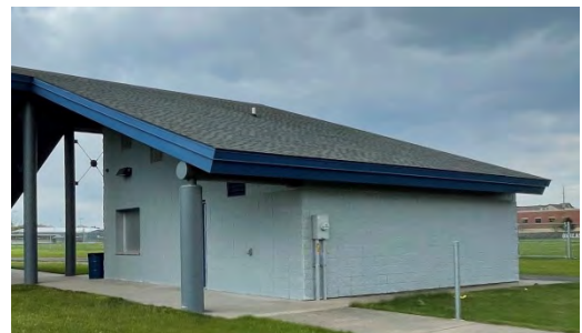
Asphalt shingled roof
