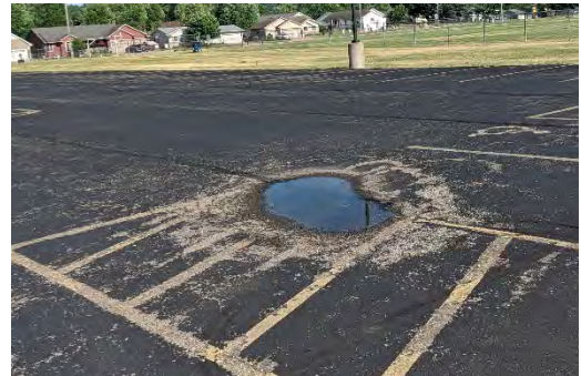
Low spot in paving – map grid I11
