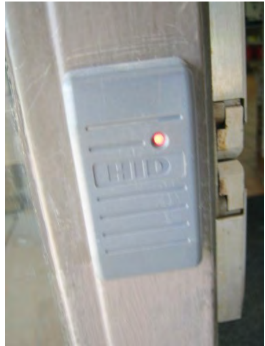
Electronic door access control device
