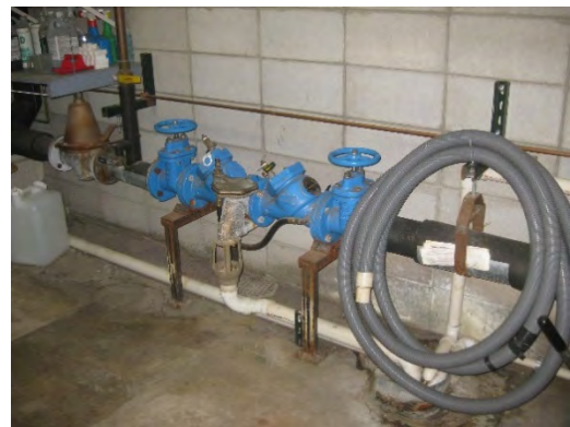
CW with backflow for HVAC chiller
