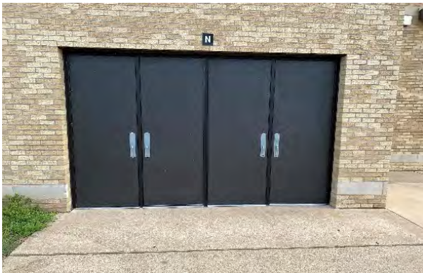
Joint seals needed – map grid D5, C6-7
