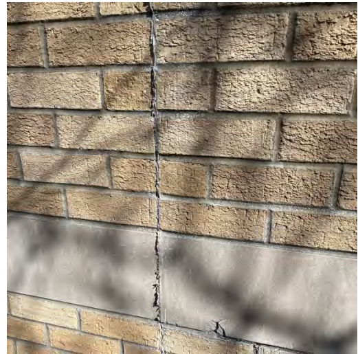
Control joint displays brick expansion
