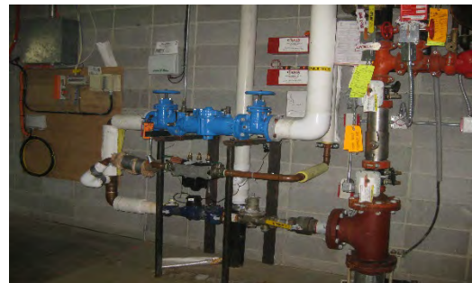
Fire protection riser, south irrigation, and CW for HVAC chiller
