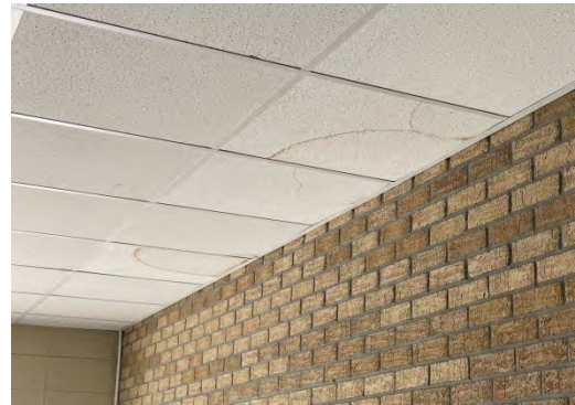
Damaged ceiling tiles to be replaced
