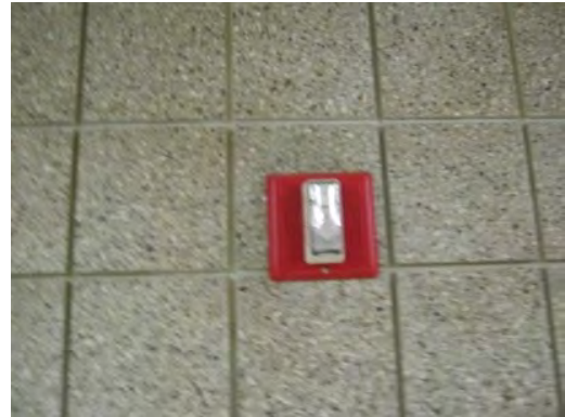
Fire alarm notification device
