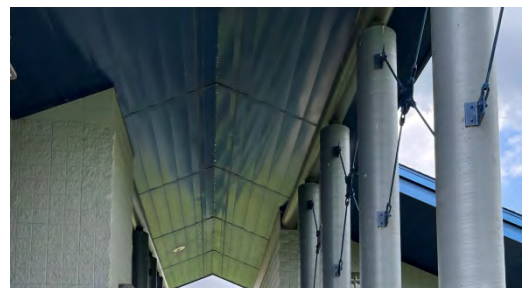
Prefinished metal soffits
