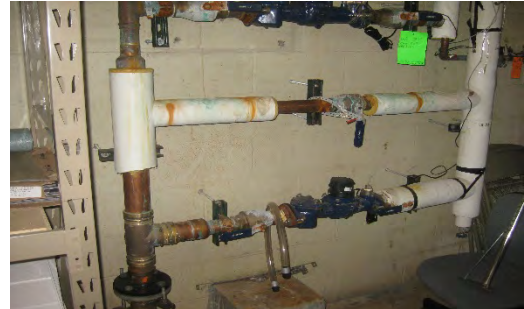
3" Domestic water service and north irrigation
