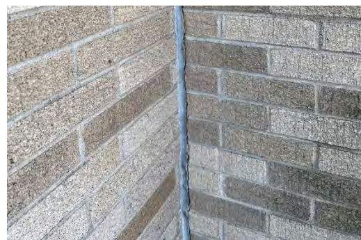
Soft joint replacement is required at various existing joints
