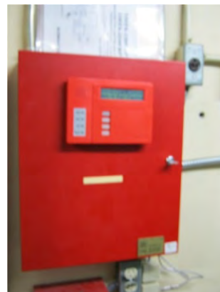
Security system keypad/control panel
