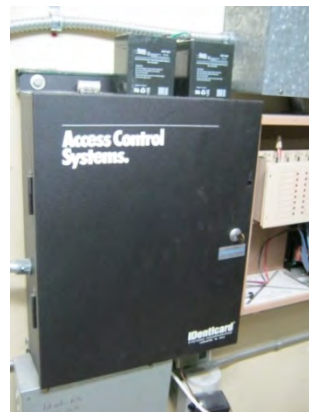
Electronic Door Access Control
