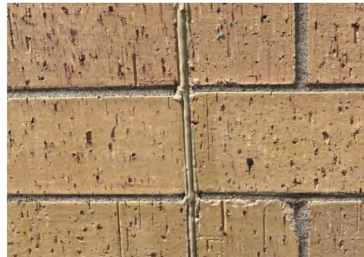
Brick expansion at gym south wall
