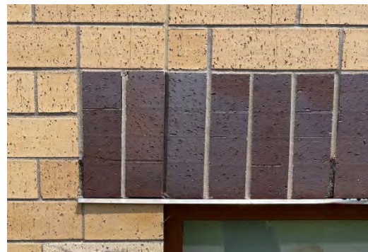
Slight movement at window lintel on left
