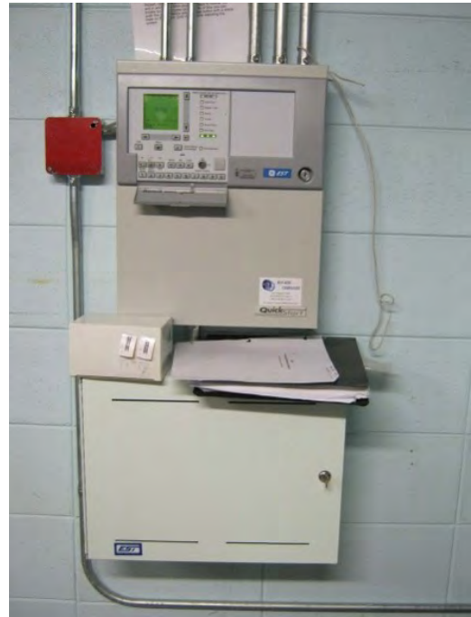
Fire alarm control panel
