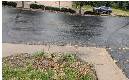
Plugged inlet – map grid G5
