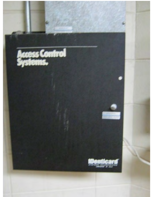
Electronic door access control
