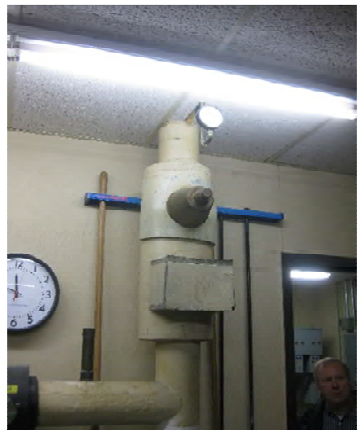
Water pressure reducing valve
