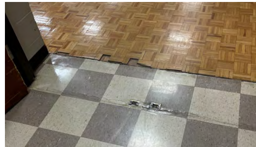
Maple gymnasium flooring and VCT display damage and cracks at threshold
