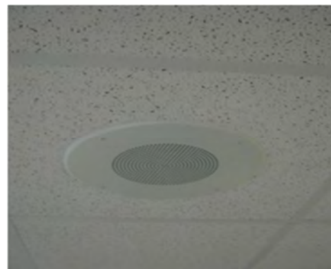
Interior public address system speaker
