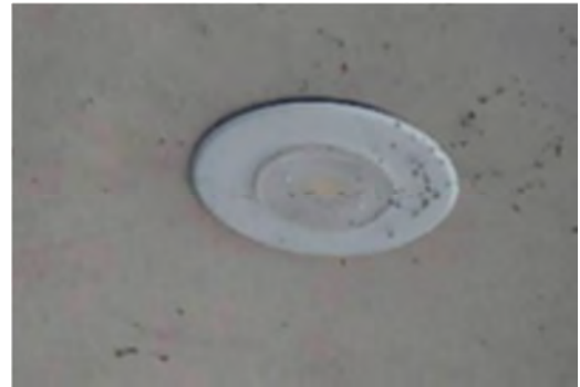
Exterior LED recessed lighting fixture
