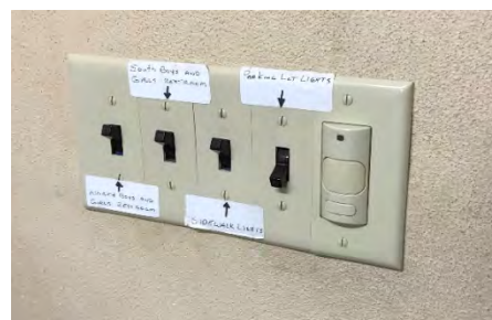
Manual exterior lighting control
