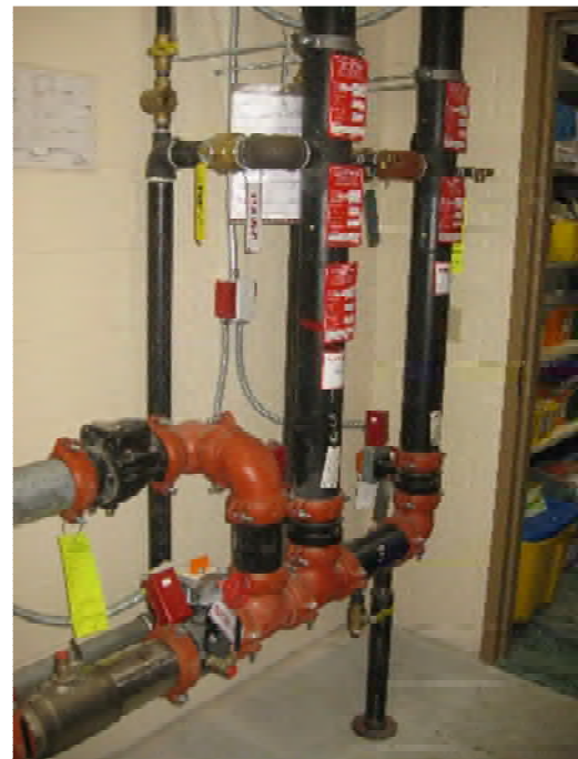
Fire protection risers (8702)
