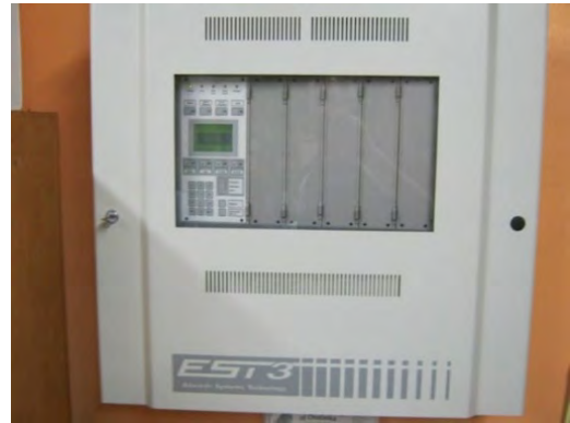
Fire alarm control panel
