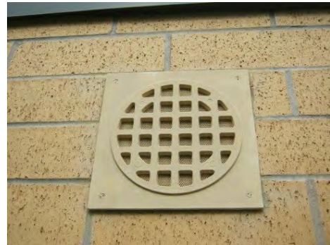
Public address system exterior speaker
