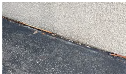
Drip flashing rusted and deteriorated
