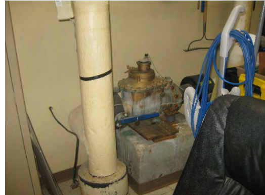
4" Domestic water service and water meter
