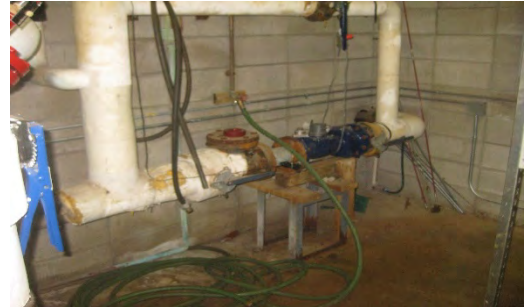
4" Domestic water service and water meter
