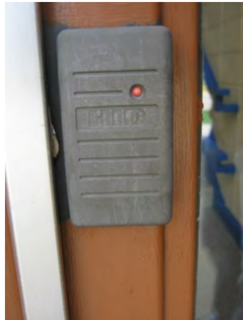
Door access system card reader
