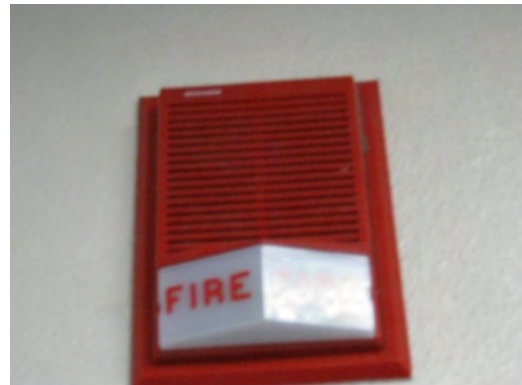
Fire alarm notification device
