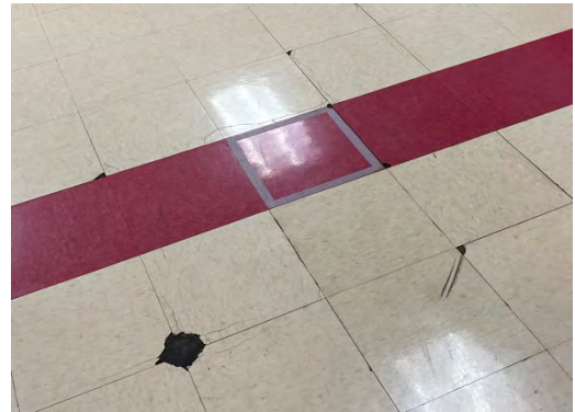
Various repairs required in resilient floors
