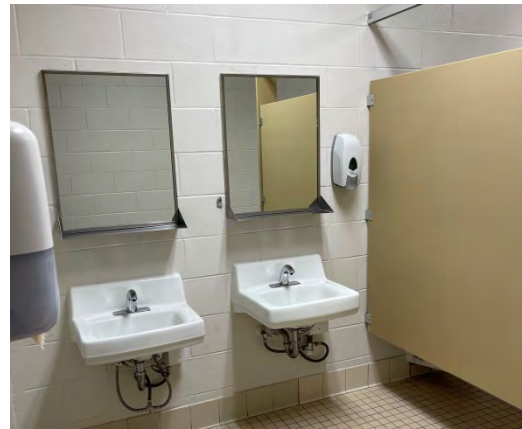
Exposed pipes at lavatories
