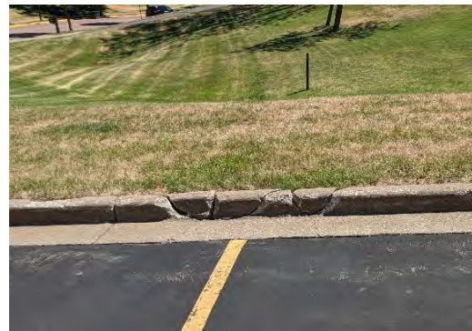
Broken curb – map grid C4
