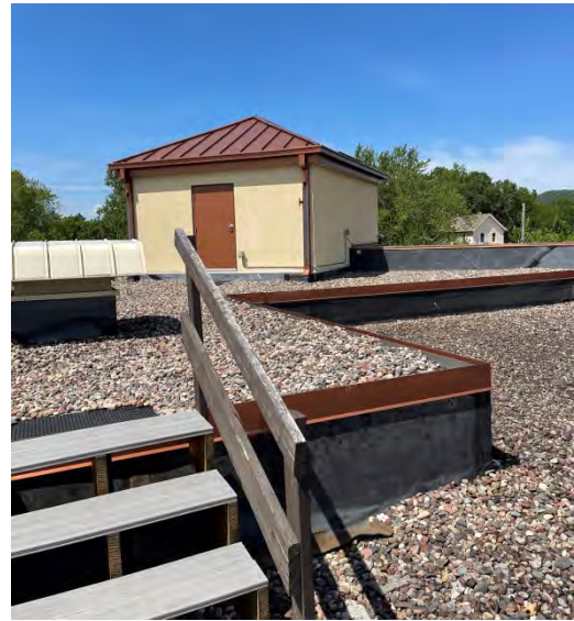
Existing ballast roof and tower
