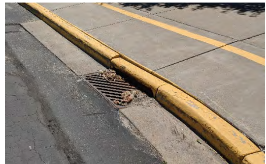
Reset curb inlet – map grid G5
