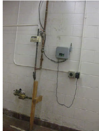
Water meter and irrigation
