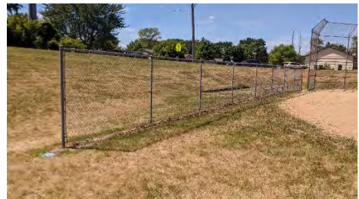
Missing end brace rail – map grid G2
