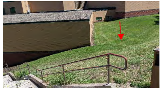
Drainage not going to inlet – map grid I3
