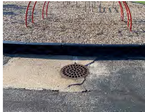
Damaged apron – map grid D3
