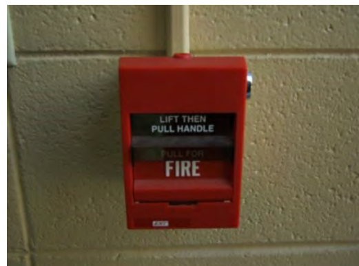
Fire alarm pull station
