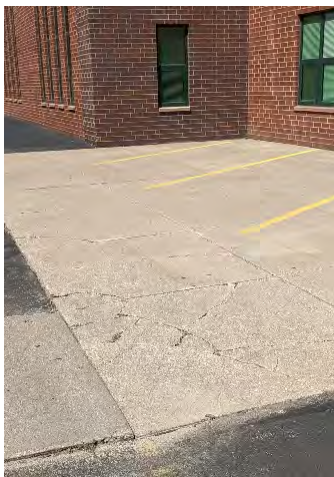
Concrete pavement failure – map grid E3
