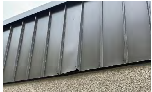
Metal ribbed panels detached
