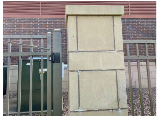
Moisture damage at mechanical enclosure
