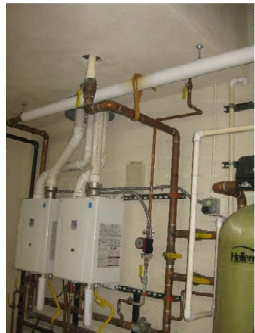
Water heaters and softener
