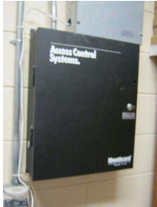
Electronic door access control system
