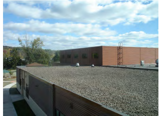
Ballasted roof at 1071 and 1991 building
