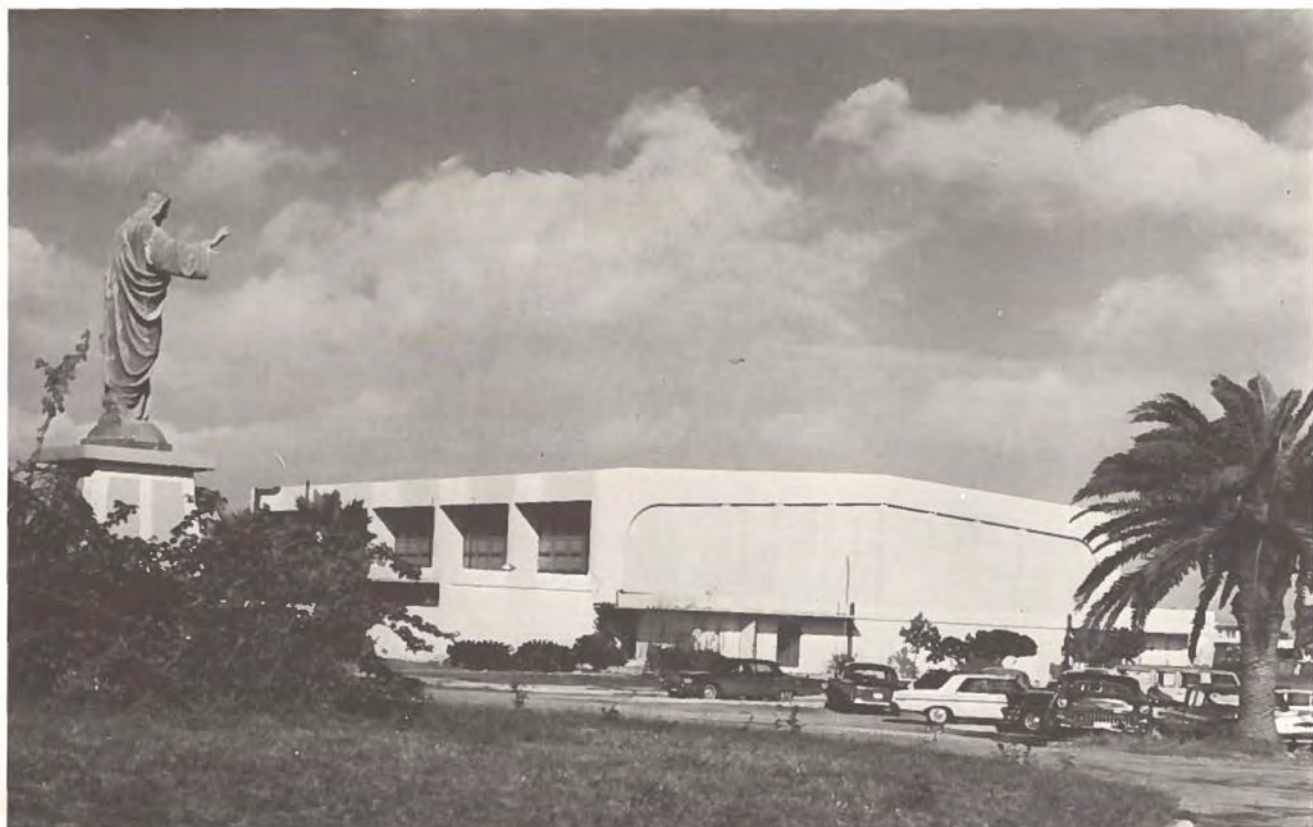
One of the outstanding high school gyms in South Texas
