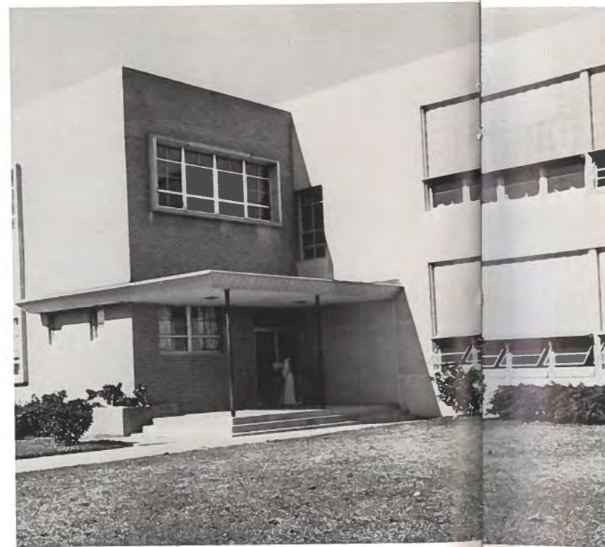
Southwest entrance to the Academy Building.
