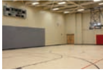
The new wood floors complete the renovation of the Sunnyside gymnasium.
