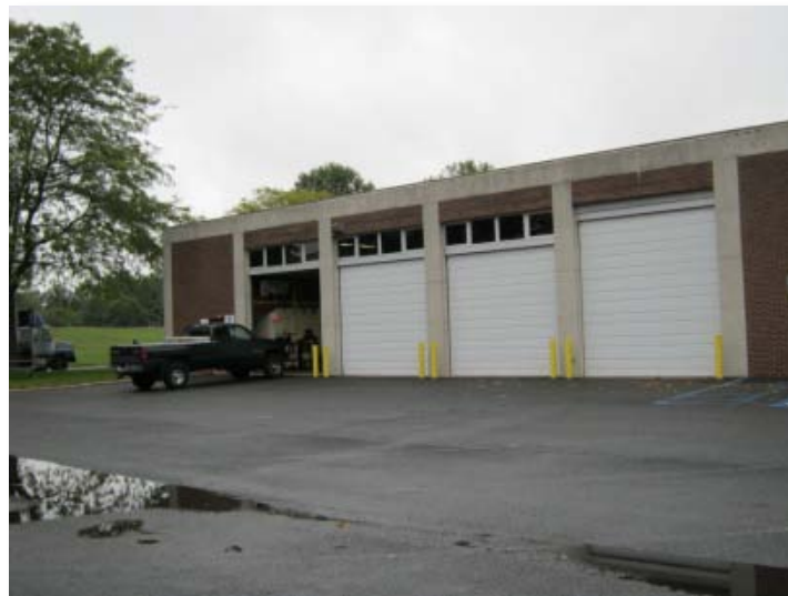
Figure 1: Garage doors at Assunpink
