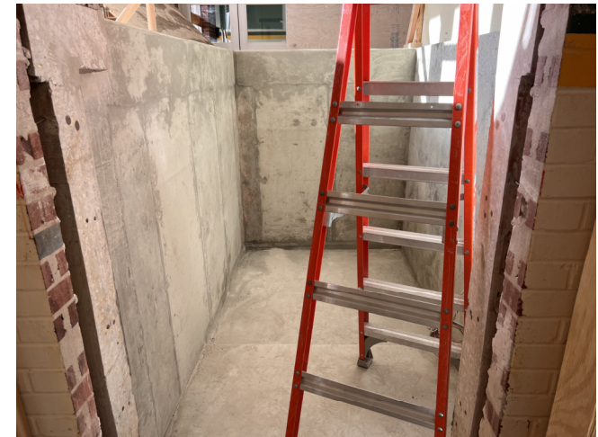
Wheelchair Lift Ready for Finishes
