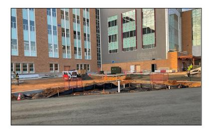
Excavation and prep for the east parking lot is ongoing. Curb and gutter installation will be completed in December, along with paving. Utility work onsite is continuing with the coordination of all new utilities serving the new building. Fire hydrant installation will be completed and testing will be executed. Exterior façade work continues on all sides of the building, including masonry installation, masonry wash down,
