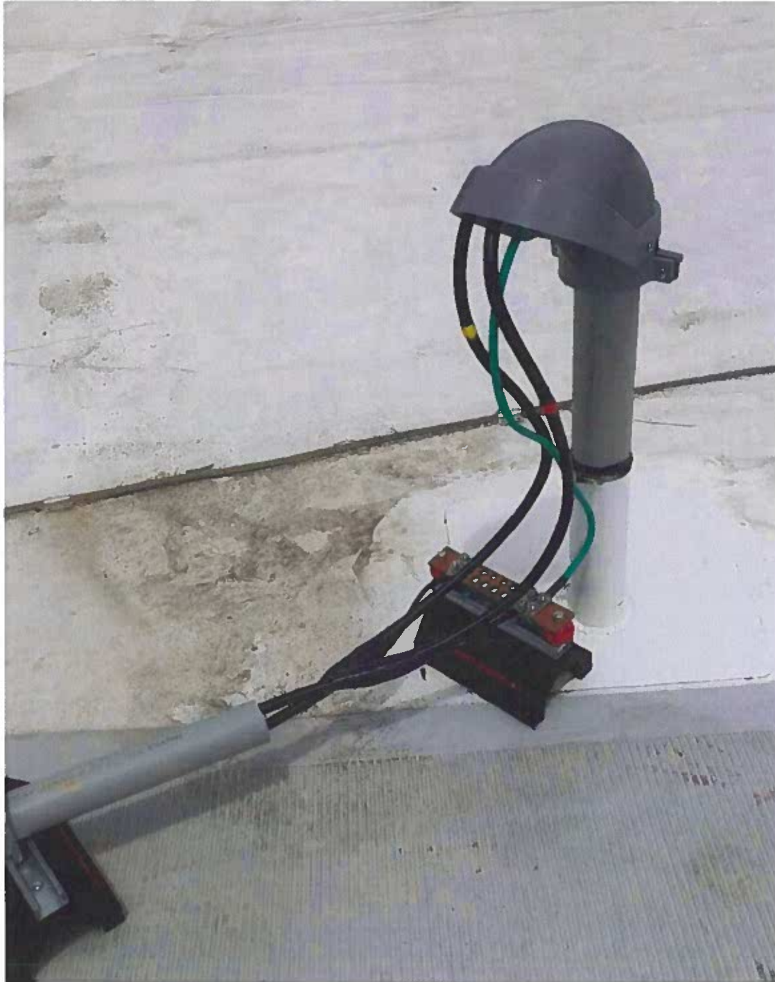
Figure 1: Photo of the Roof Penetration that will be used to connect the GPS antenna to the Small Cells.
