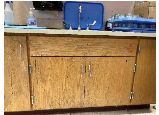
3.13 Damaged classroom casework and hardware.
