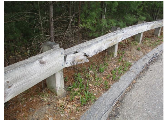
1.7 Damaged timber guardrail.
