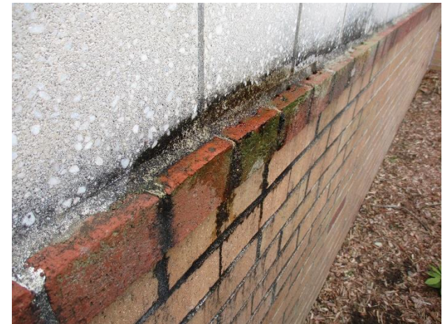
2.14 Water infiltration at ground face block by the gym.
