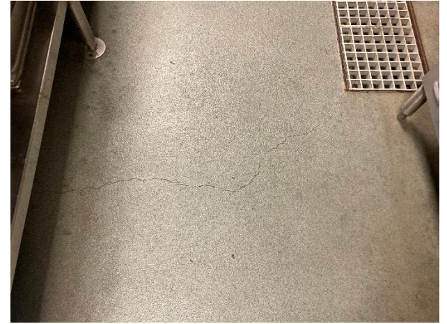
3.7 Cracks in epoxy flooring in kitchen.
