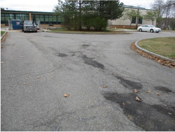
1.1 Slight bituminous deterioration at driveway.
