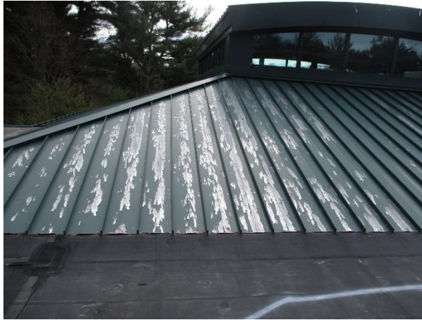
2.3 Deteriorating standing seam metal roof system.
