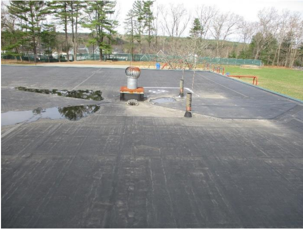
2.1 Ponding near roof drain.
