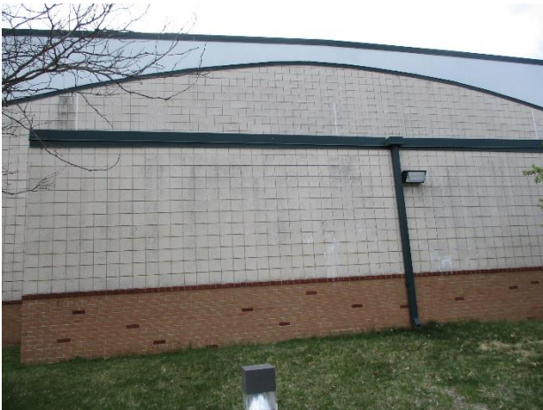
2.8 Staining and efflorescence at ground face blocks.
