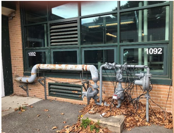
4.21 Corroded exterior gas piping.
