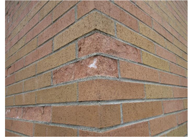
2.6 Cracked and spalling bricks.
