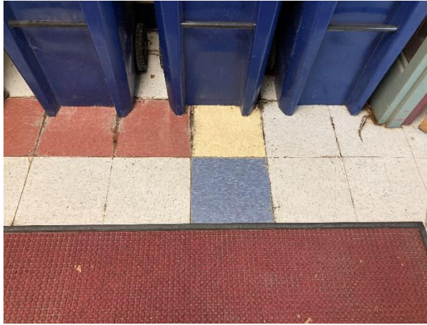
3.4 Water infiltrating and deteriorating VCT flooring in corridor.
