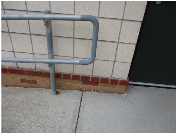
1.6 Handrail extension does not meet ADA requirement.
