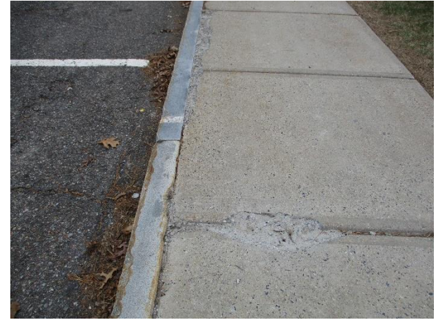
1.4 Small area of deterioration at the concrete sidewalk.
