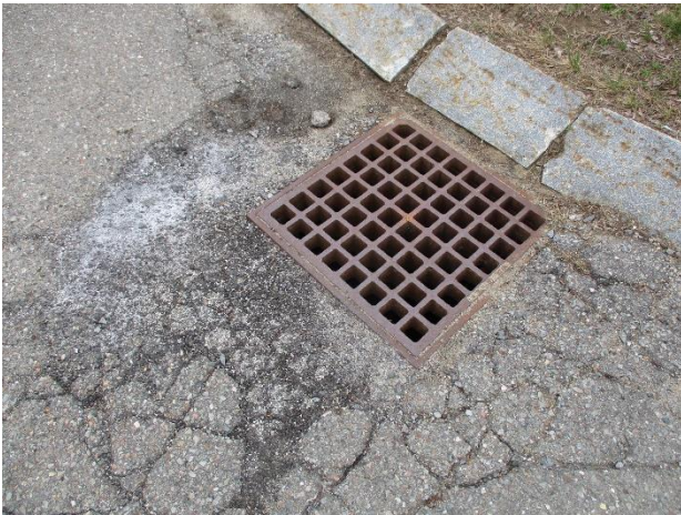
1.5 Settling storm drain and deterioration of bituminous pavement.
