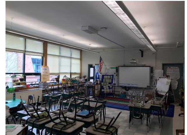
5.1 Suspended fluorescent light fixtures in classroom.
