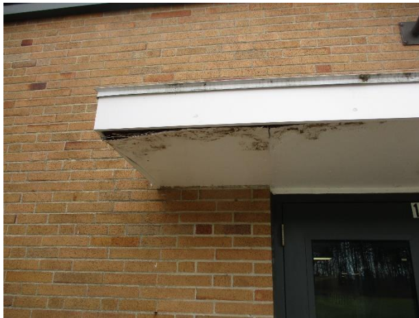
2.11 Deteriorated soffit by Door #10.
