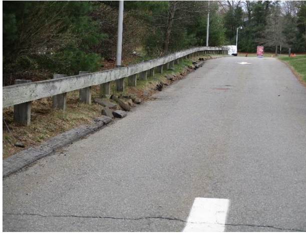
1.2 Damaged bituminous curbs.
