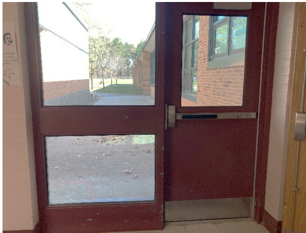
3.12 Corroded and peeling hollow metal door and frame.
