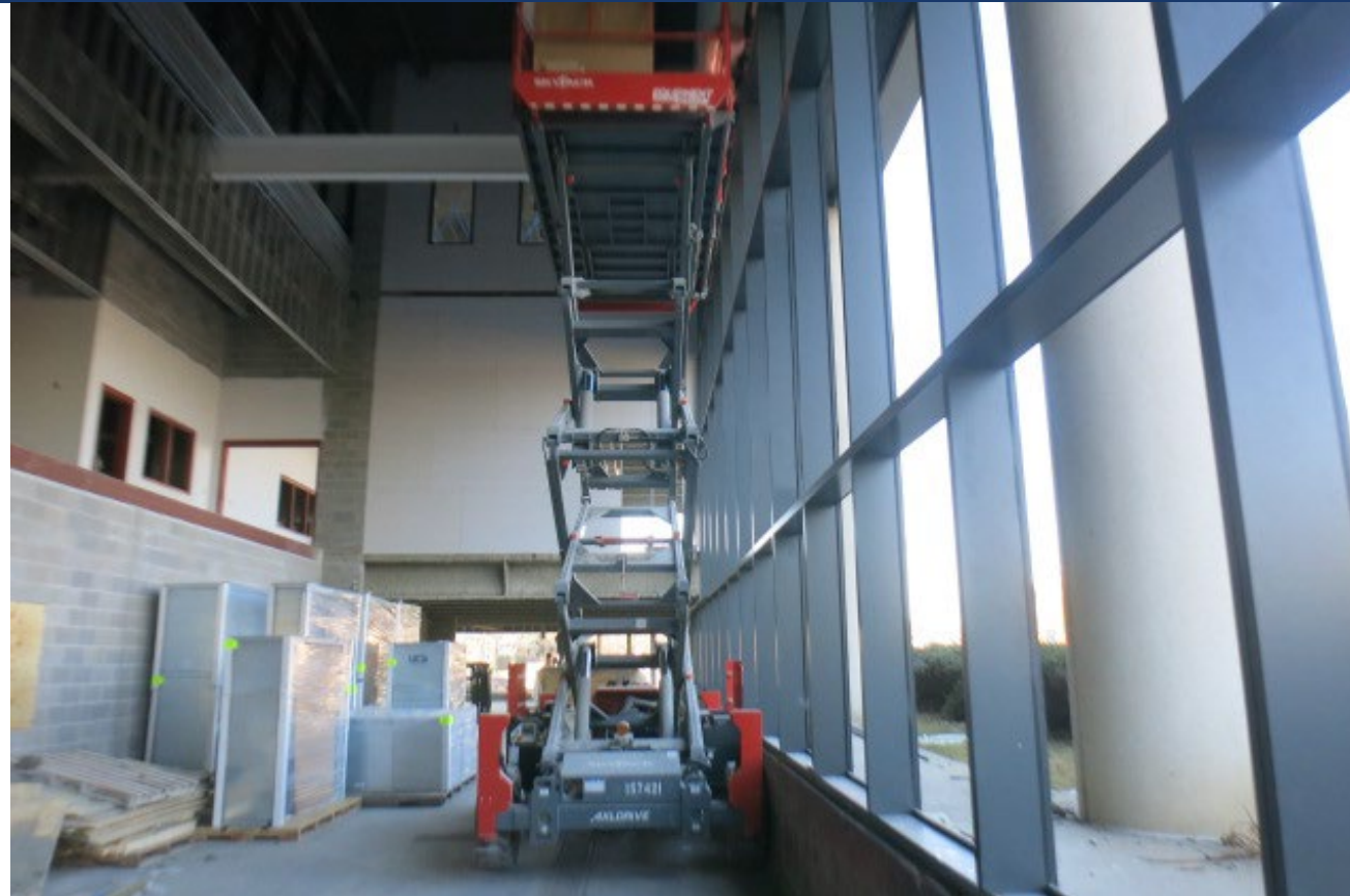
Curtainwall framing continuing
