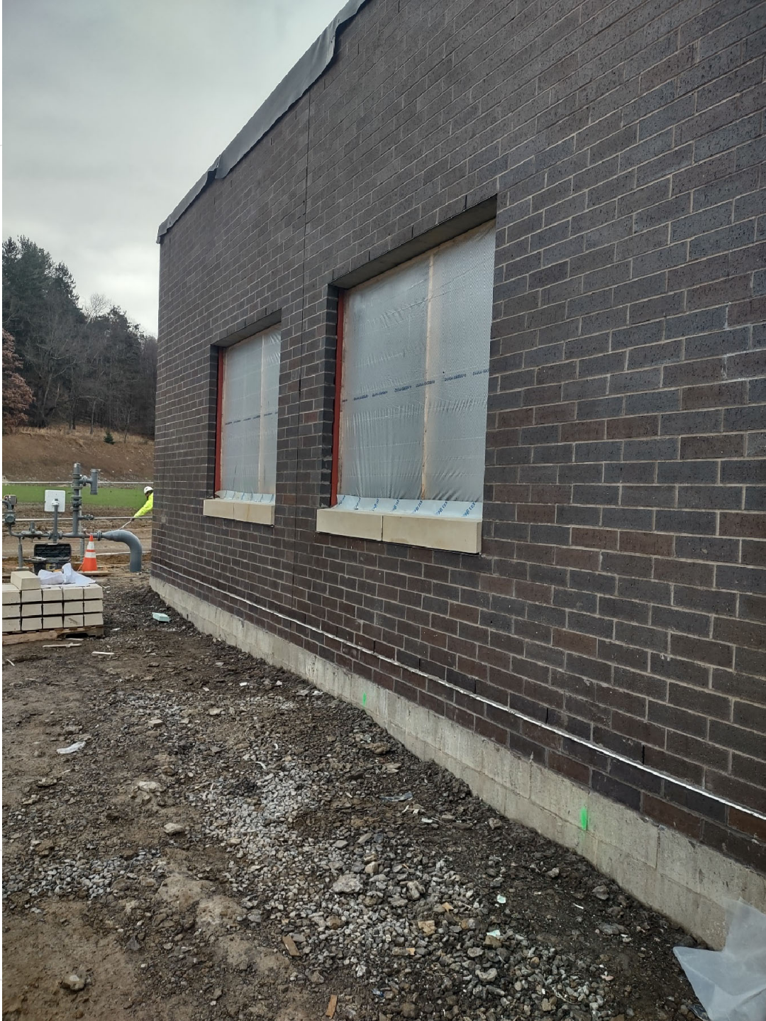
Northwest corner of Area A Addition with sills installed and scaffolding removed
