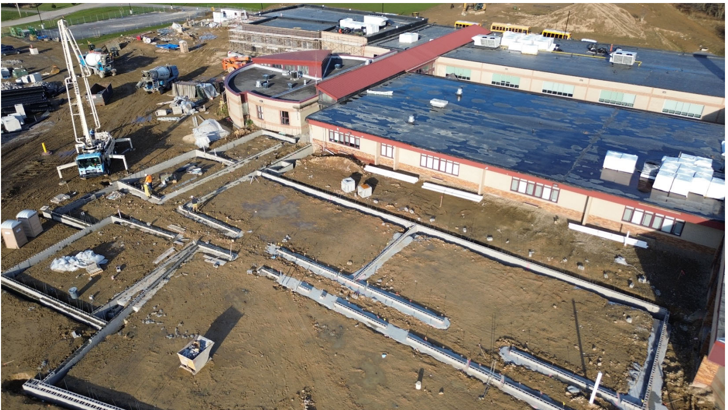
Area C Foundations in place. Classrooms closest to existing building, administrative/office area in foreground.
