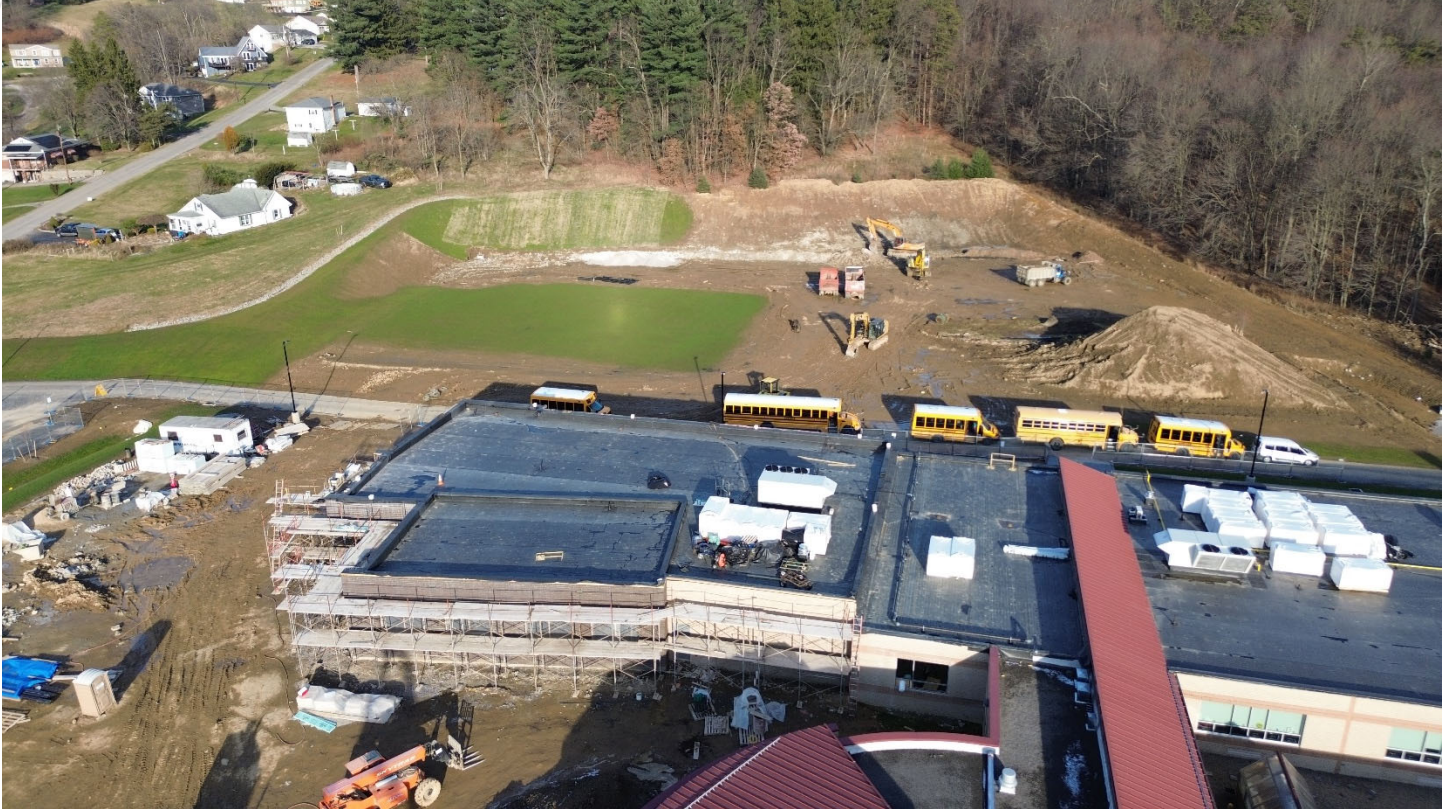
Athletic field final grading well underway. Underdrains being installed at toe of slope to the north side. Busses lined up at temporary student entrance.
