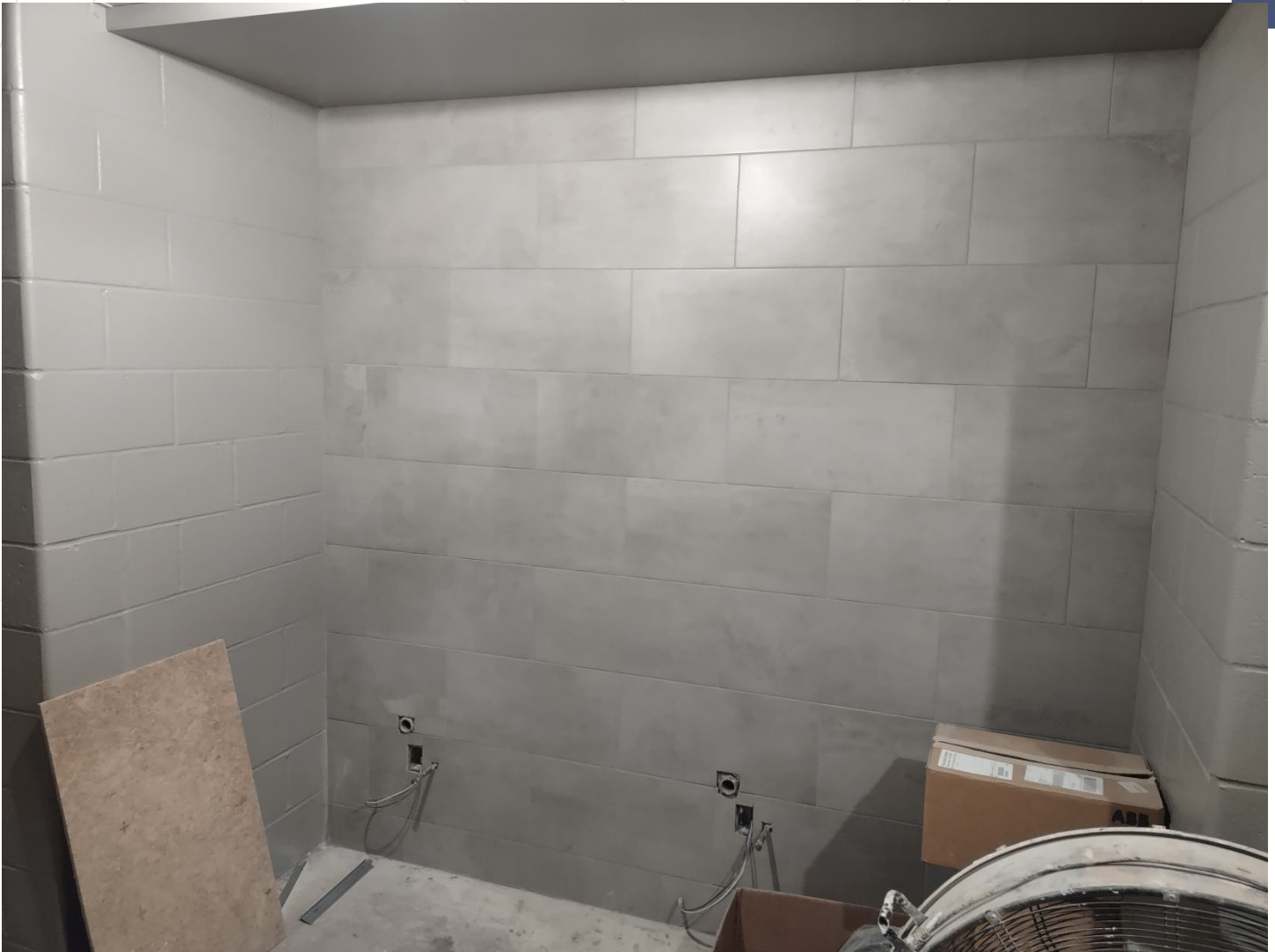
Area A Addition Restroom wall tile installed.
