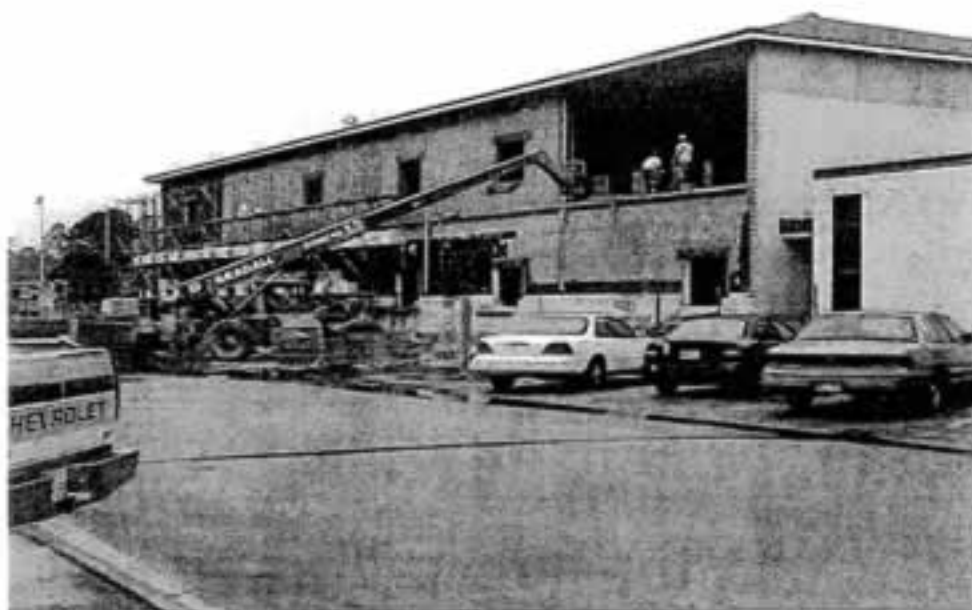
Construction underway at A. M. Barbe High School
