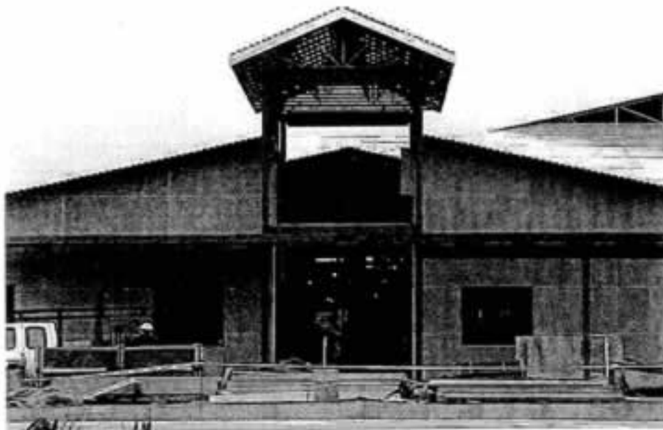
Construction underway for the new St. John Elementary School
