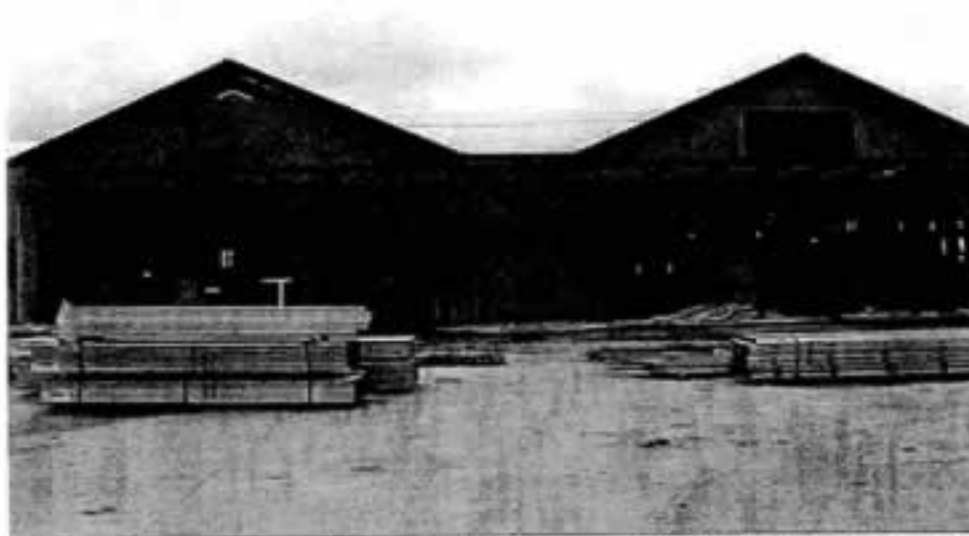
Additional construction underway for the new St. John Elementary School
