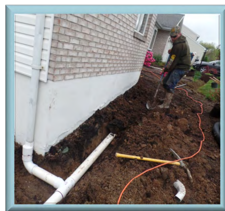
Austin Schwenk covers drainage pipe he installed for Silver Maple Landscaping in Orwigsburg.
