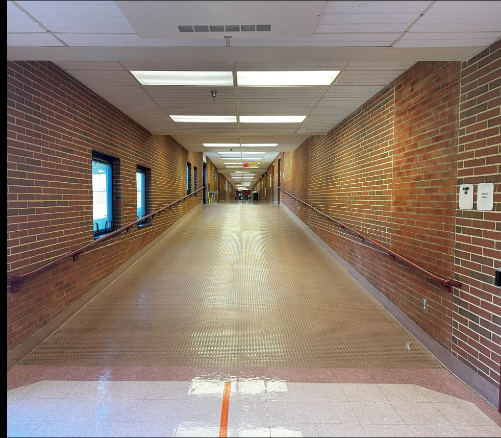
Existing ramp does not meet ADA accessibility
